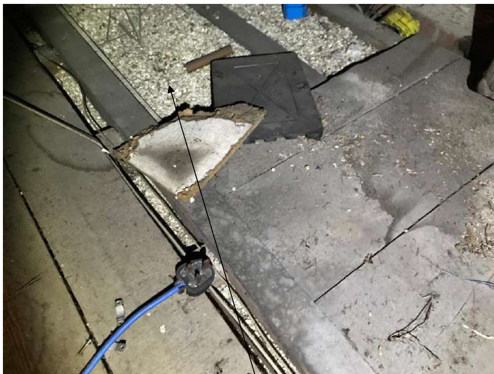
Loose Fill Insulation
