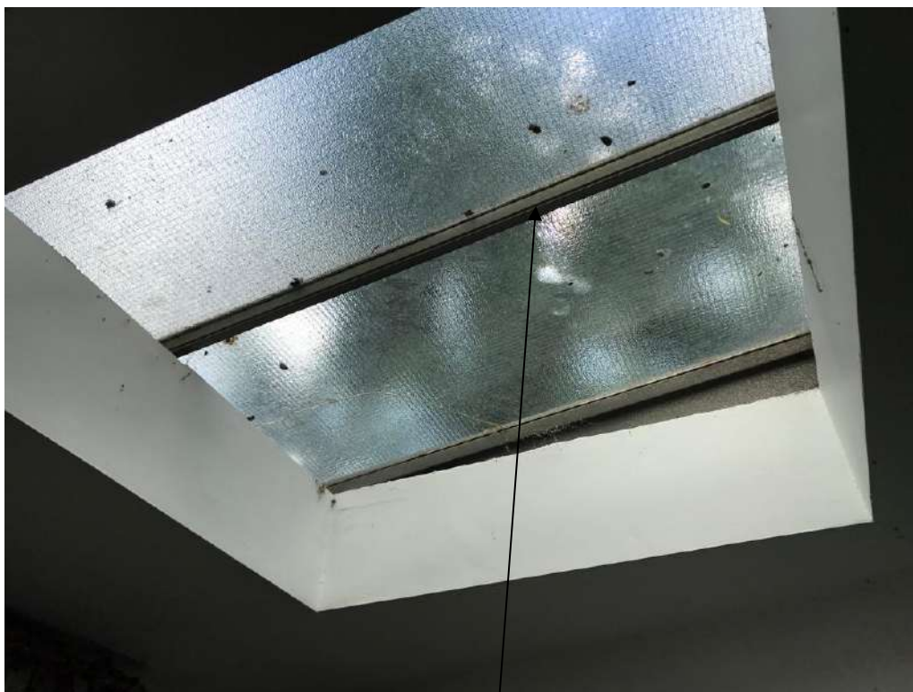
Rope Gasket to Skylight
