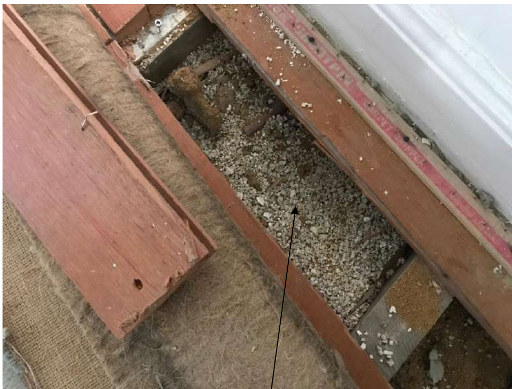
Under Floor Insulation
