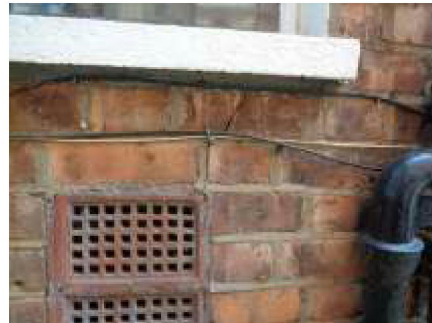
Cracking to the left elevation below the foremost window
