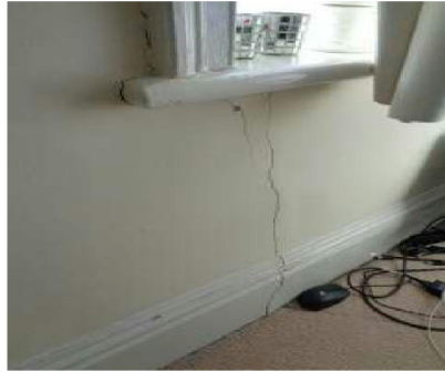
Cracking beneath the front window in flat 3
