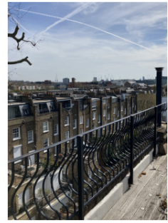
Fig 11 : Fourth floor terrace view facing E
