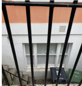
Fig 14 : The basement front lightwell
