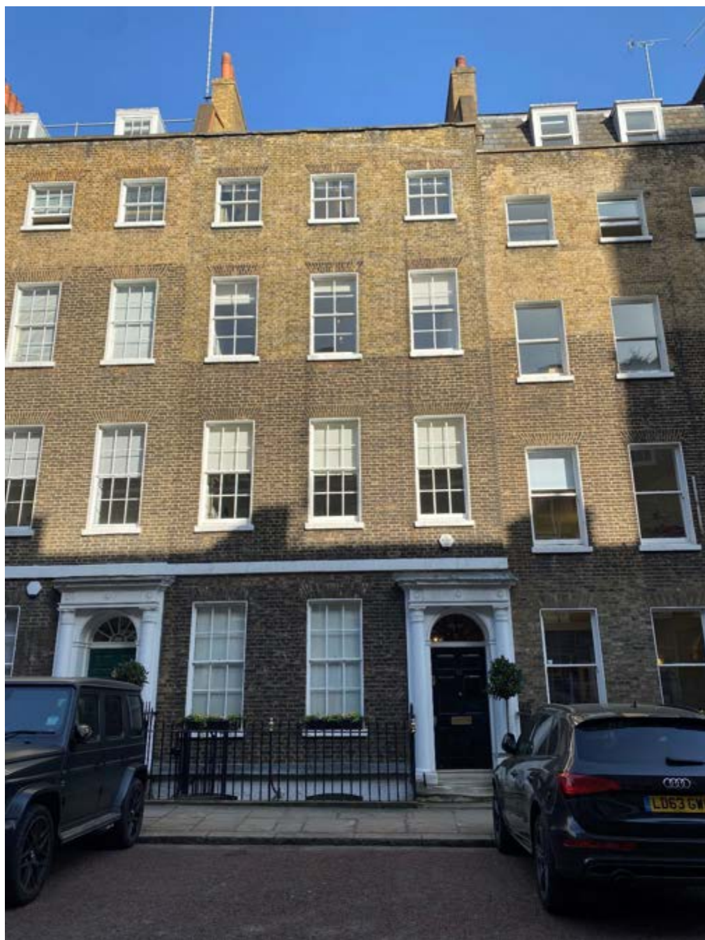
Photo of front elevation of 33 Ely Place
