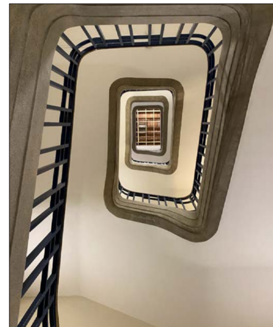
Fig. B Gower Street stairwell - view from Ground level looking up
