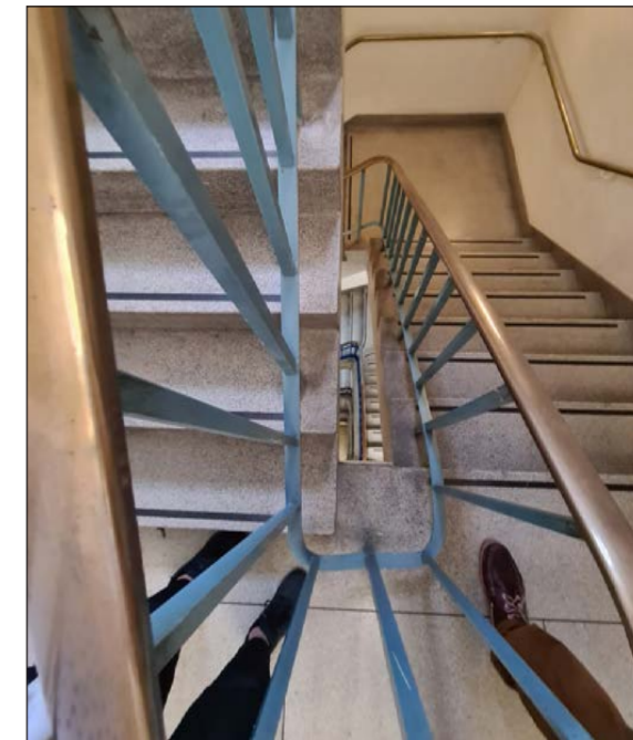
Malet Street stairwell - view from top storey landing looking down
