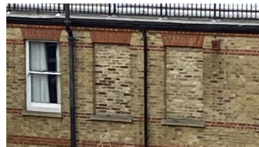
Examples of other bricked up windows in the north courtyard
