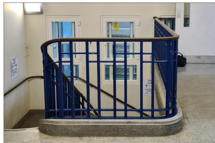
Existing balustrade at level 4
