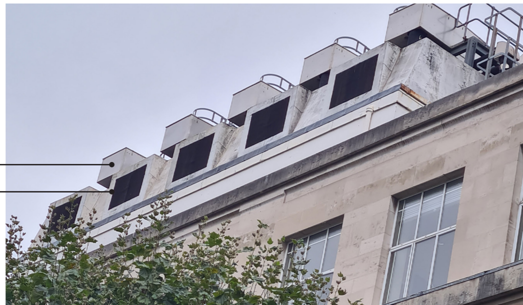
Existing photo of Gower Street Mansard Roof
