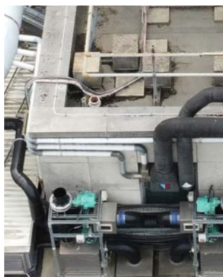
Existing condition of parapet
