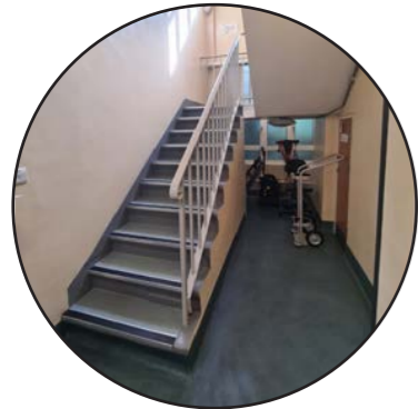
Stair between L4-5 to be demolished
