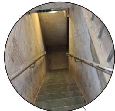
Fire escape between L4-5 to be demolished
