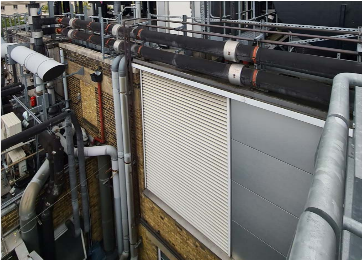
North facing louvered facade to Plant Room on Level 5
