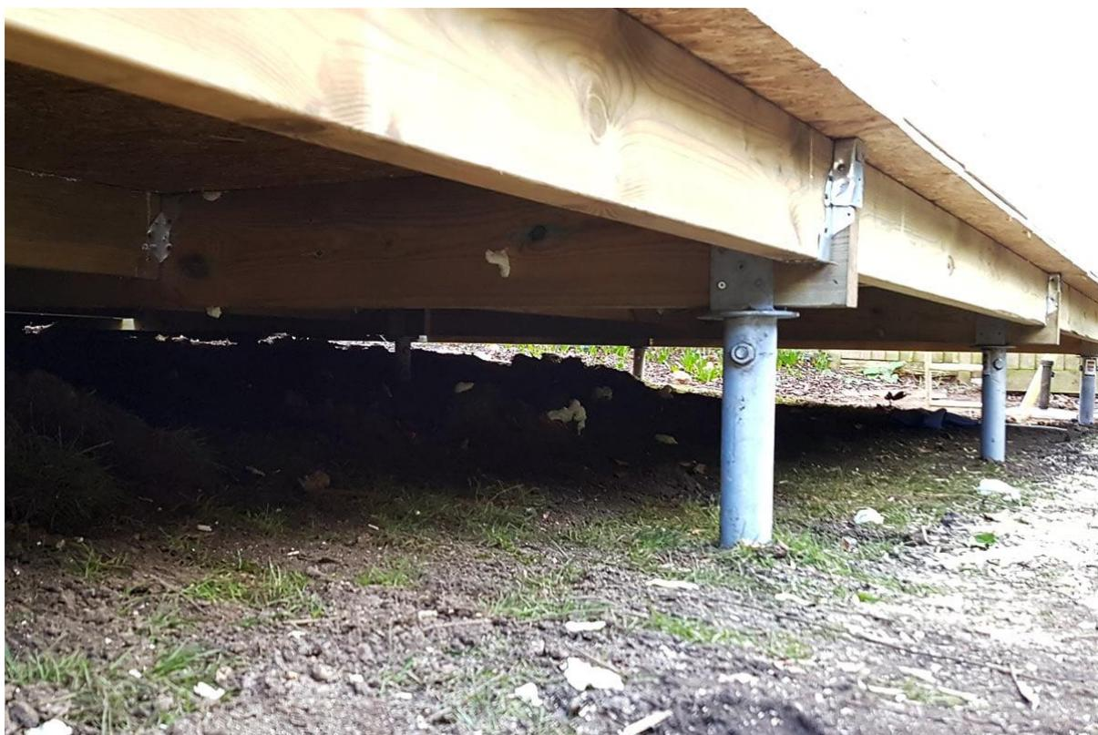
**Photograph 5:** Screw pile foundation with void beneath building.
