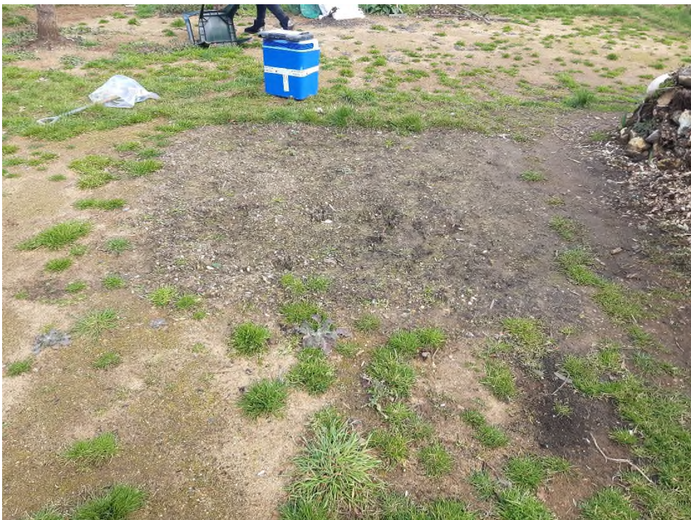
Plate 2: VISIT 27/02/23 View of plot 19b looking south focusing on area that has been further remediated .
