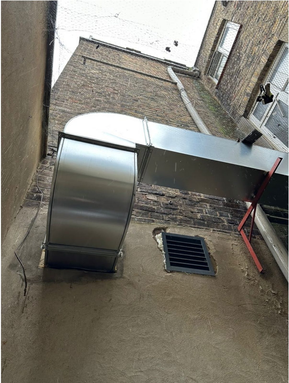
Photo 2 View of exhaust ductwork penetrating the facade
