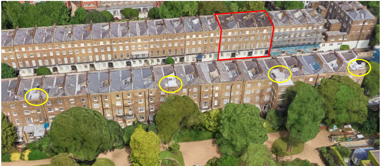
Figure 2 – Existing lift overruns (marked in yellow) set discreetly in the valley roofs of the neighbouring hotels at 24-27, 31-32, 34-37 and 39-40 Bedford Place with Site marked in red.
