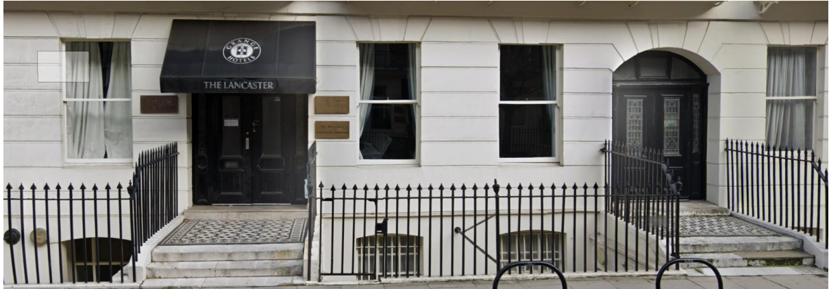
Figure 1 – Entrance to Hotel.
