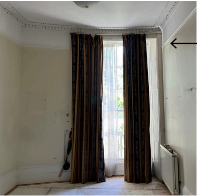
Although these partitions appear to be of an age & contain some original features they are not considered original. Partitions therefore to be removed and curved apsidal wall to be reinstalled in No's 4 & 6.
