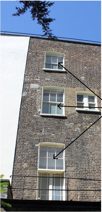
LOCATION A - Windows would be retained with mirror fixed behind to conceal lift shaft.
