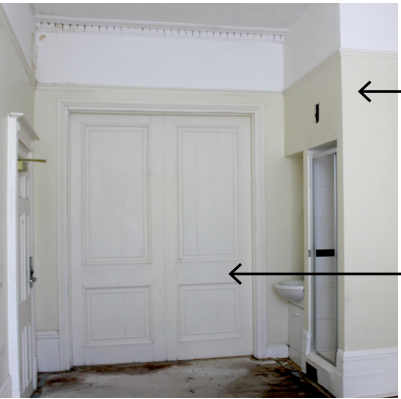
Modern partitions including bathrooms removed
