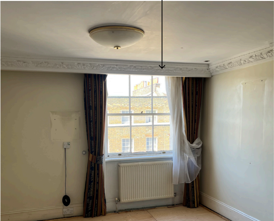
Non - original dropped ceiling evident, overlapping the existing windows and potentially hiding original features
