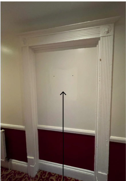
Several existing doorways have been in-filled, removed or relocated throughout the building.
