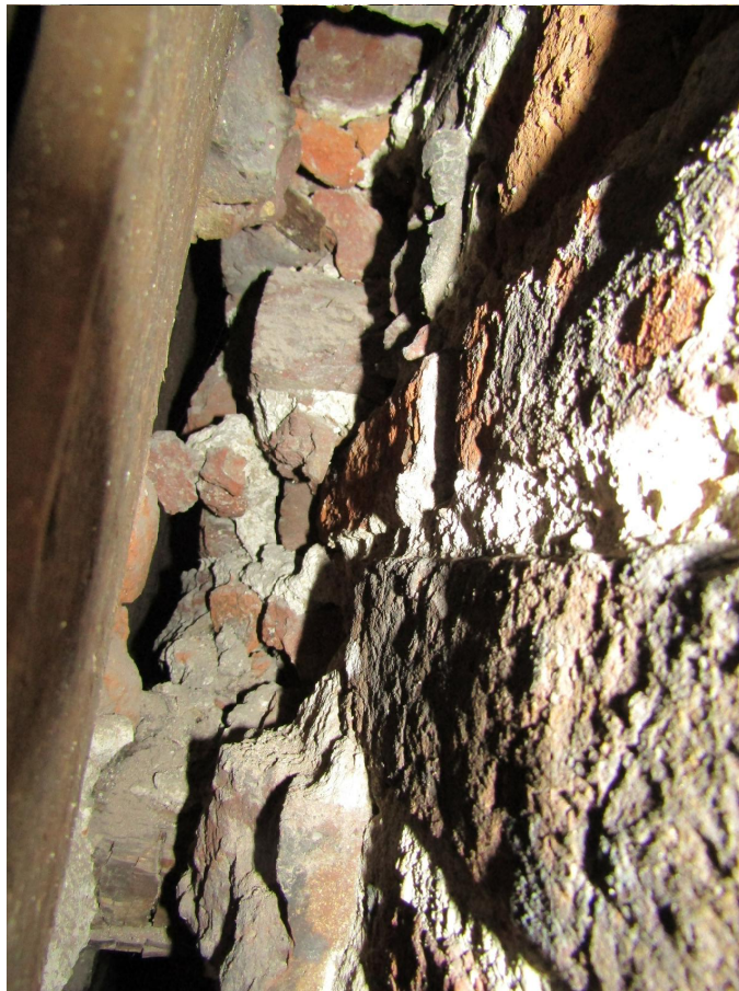
Plate 6 – Crack damage to chimney stack
