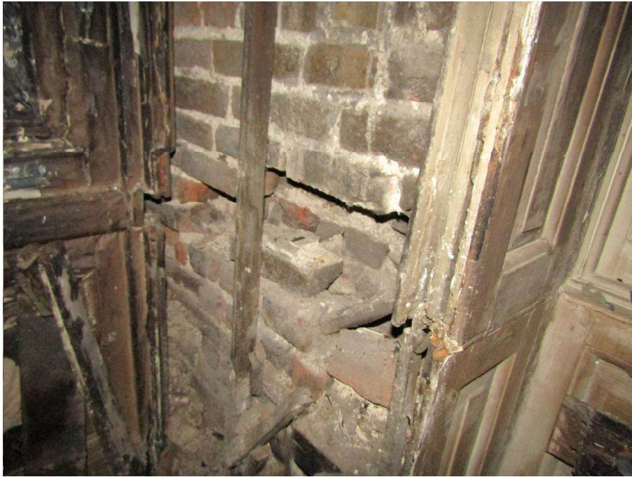
Plate 5 – Front wall void
