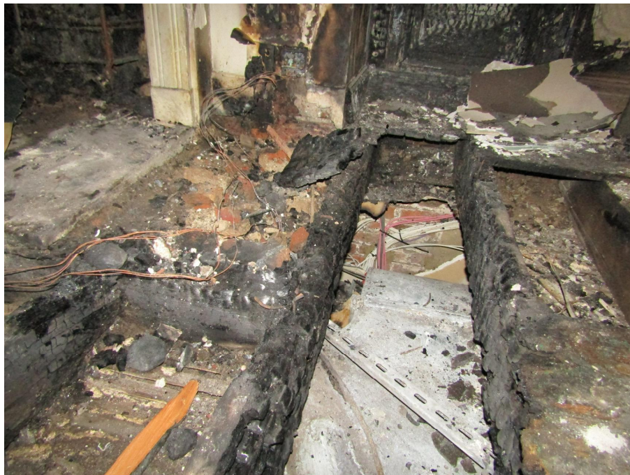
Plate 4 – Charring to chimney trimming and floor joists
