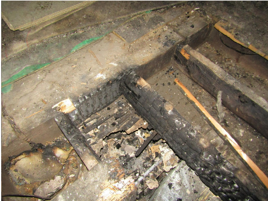
Plate 3 – Charring to main floor beam and chimney trimmer
