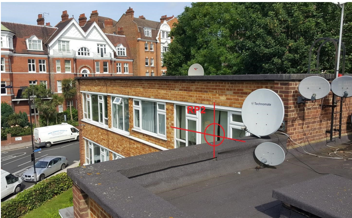
2: Second floor living room window in foreground (RP2)
