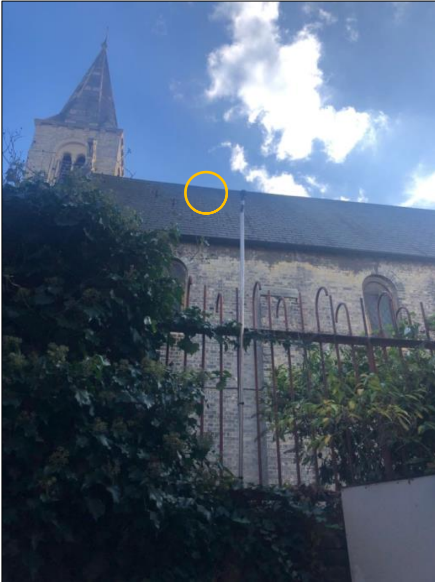
Figure A.2: Photograph of Location NM2
