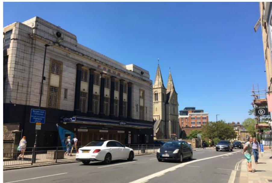
Figure 19: The Forum, Grade II, blocks longer distance views of the church, so that the church instead becomes gradually revealed as part of a series of views moving northwards along Highgate Road.
