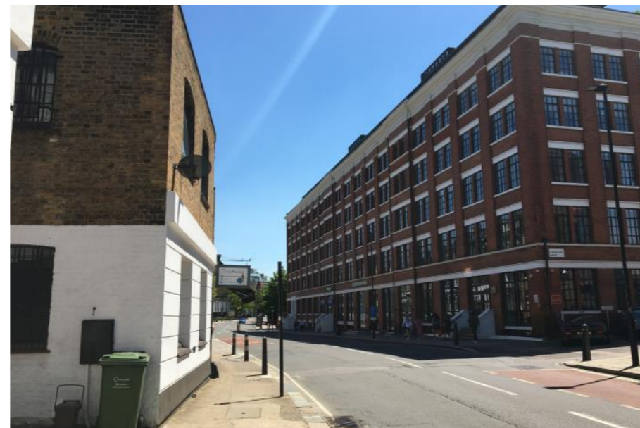
Figure 23: Views from the conservation area towards the Site are restricted by tall former industrial buildings on Highgate Road and the curve of the road.
