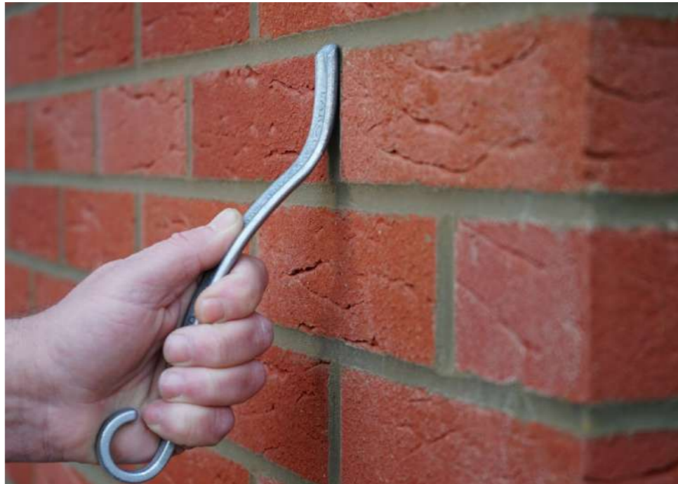
BUCKET HANDLE MORTAR JOINT
