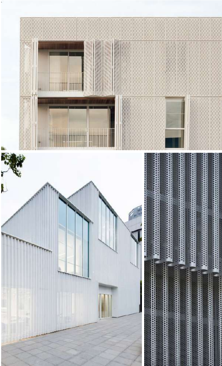
1. Base: Perforated 'veil', clearly broken at entrances, lit up by spaces behind, drawing on local industrial characteristics, re-interpreting the glazed base of the local vernacular style.
