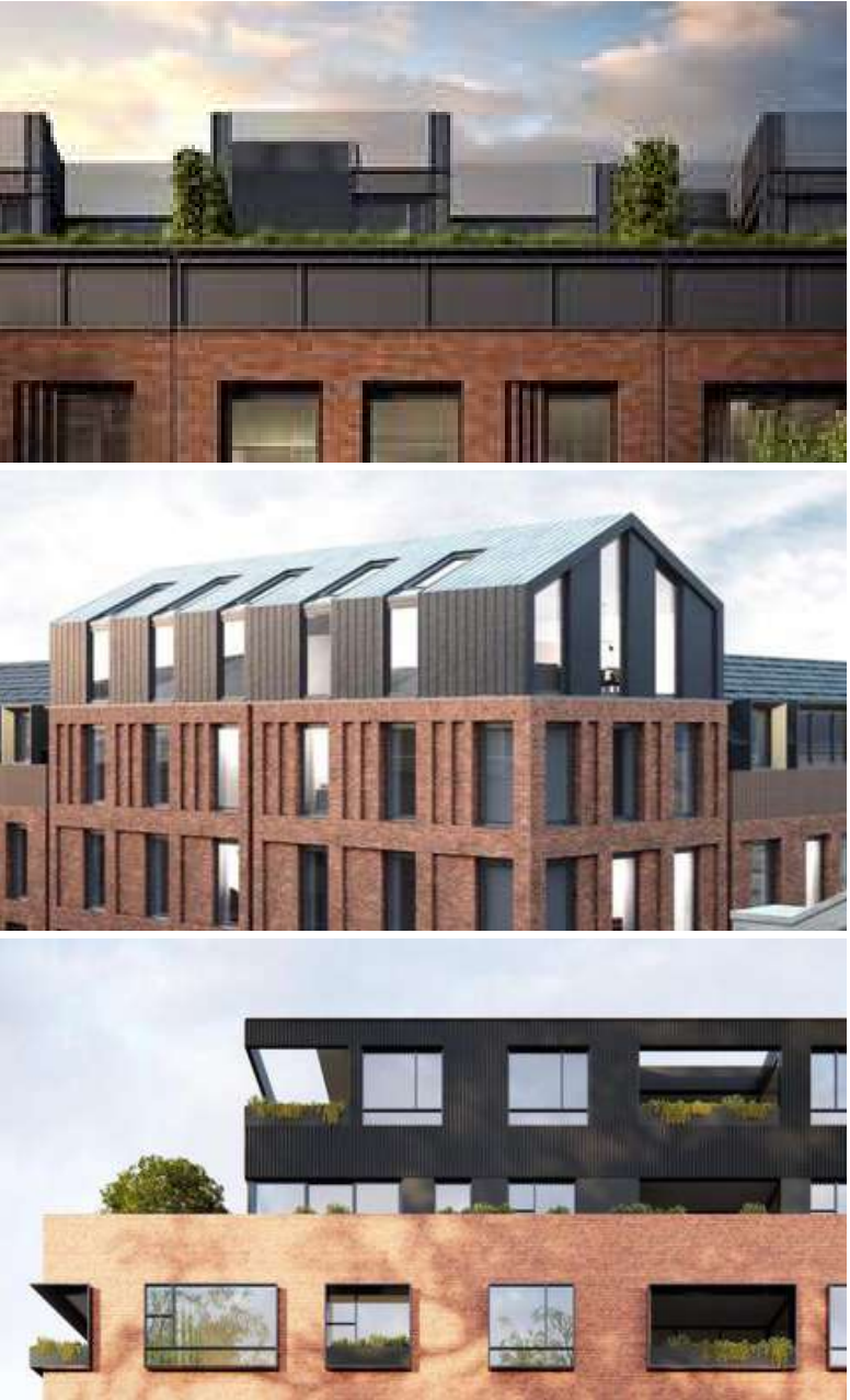
3. Top: Set back and clad in metal, re-interpreting the mansard roof, with the addition of greenery breaking-up the 'grey line' in a similar manner to the Victorian/Edwardian roofing and chimney details.
