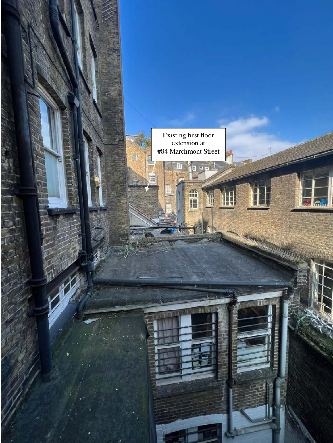
View of first floor extension at neighbouring # 84 Marchmont Street
