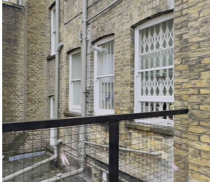
Photo 1. Rear elevation of 82 Marchmont Street, kitchen served by two nearest windows
