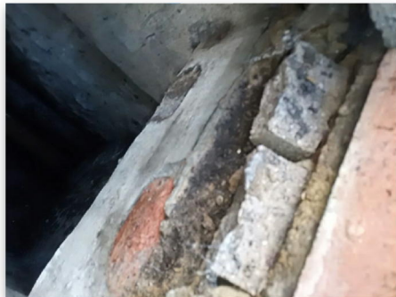
Fig 3.2: Defective MH1 chamber walls
