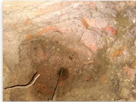
Fig 1.2: Trial Hole 1 Footing
