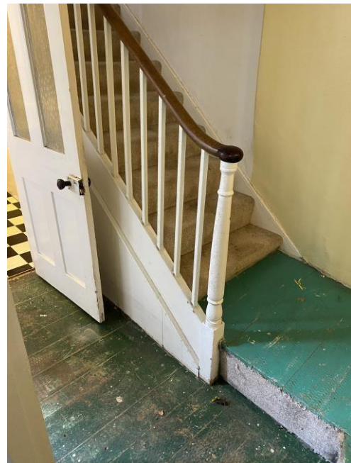
Figure 17: Original stair with bottom step altered from LGF.
