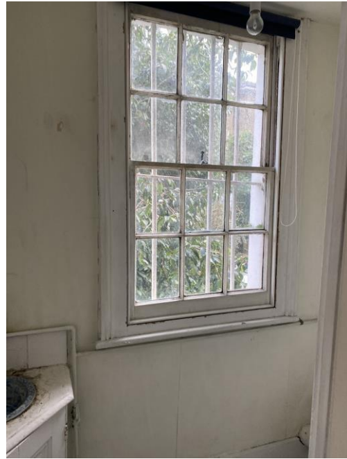
Figure 16: Original window to rear bathroom.
