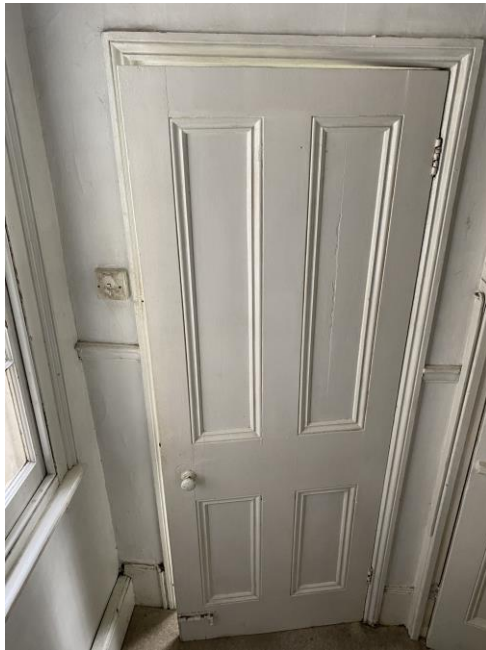
Figure 15: Door to rear bathroom with moulded detail to panels on the house side and simple four panels on the inside.
