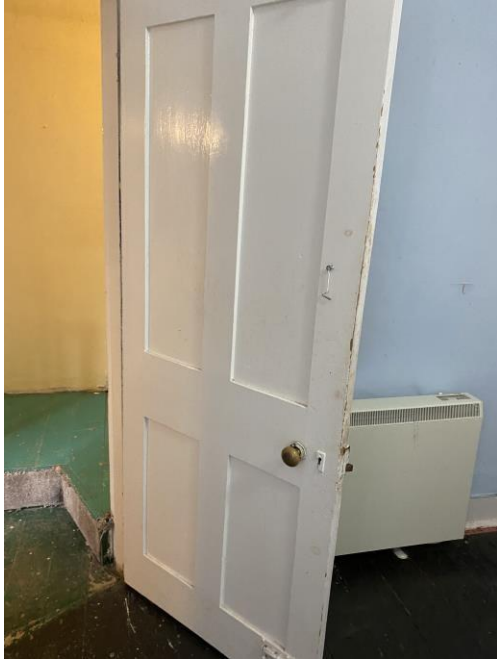
Figure 24: Door to rear room with typical details
