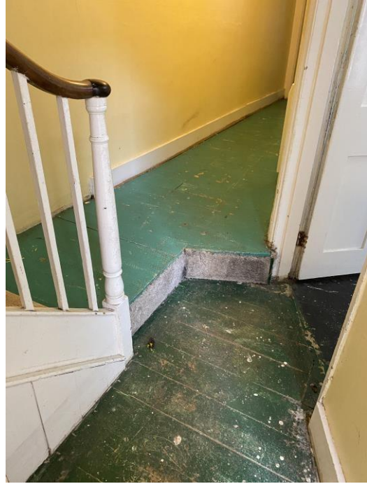
Figure 20: Platform in lower ground floor hallway.
