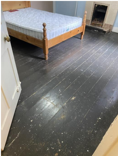
Figure 25: Rear room floor finish.
