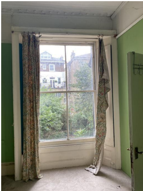
Figure 12: Rear room window with lining and shutters.
