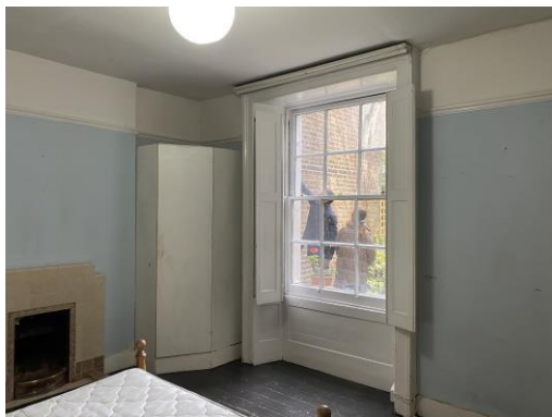
Figure 22: Rear window to rear room and 1930s style fireplace.
