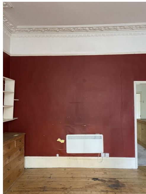
Figure 11: Partition to rear room with non-original door opening.
