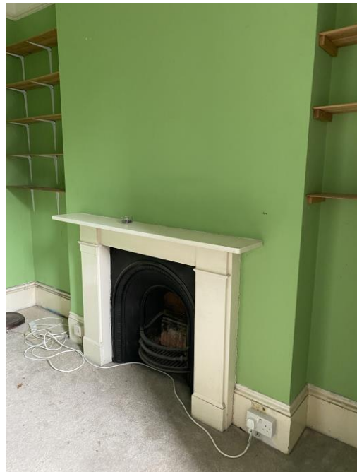
Figure 14: Original fireplace to rear room and original skirting.
