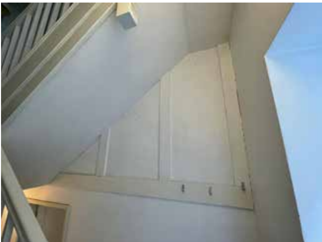
[Fig. 10] Panelling to stairwell, to be removed.
