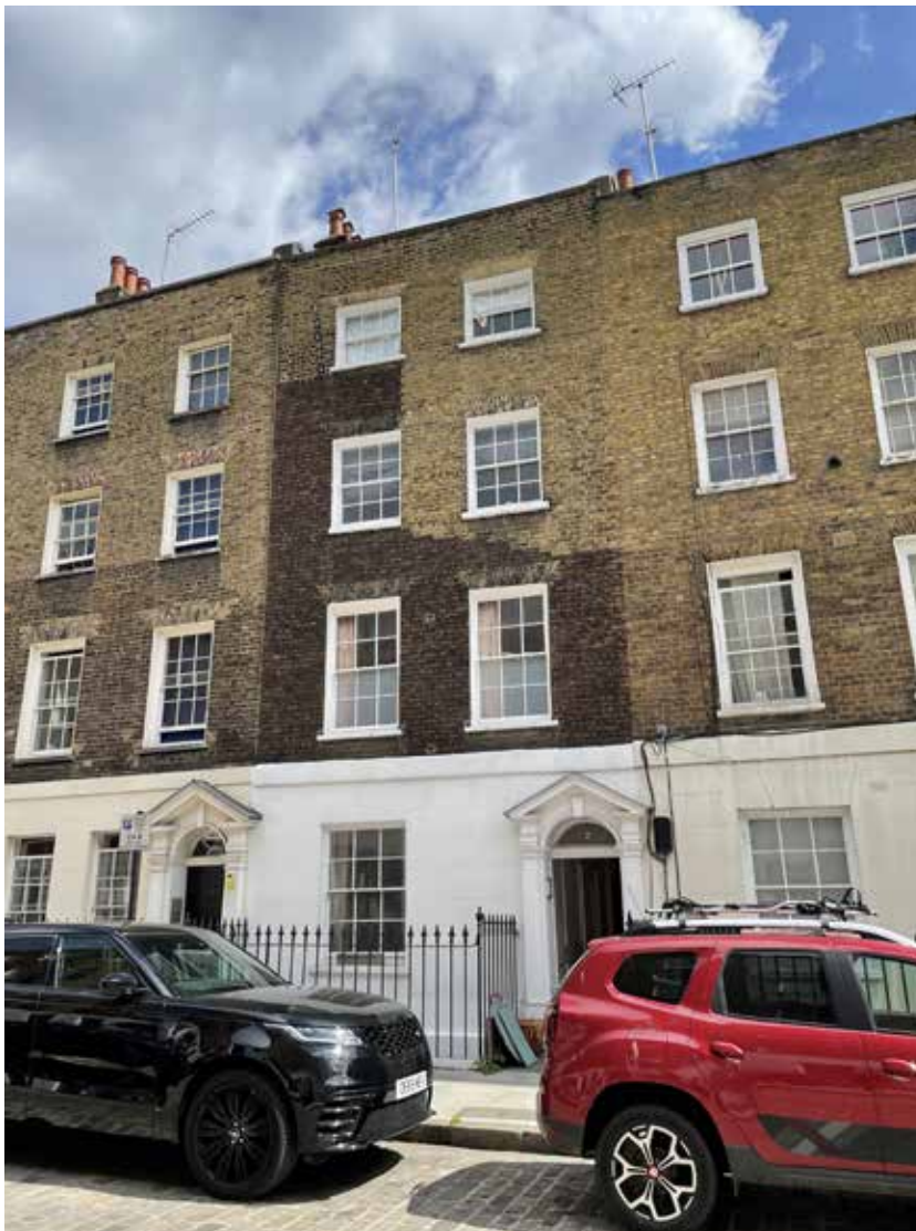
[Fig. 01] View of front of property as existing.
