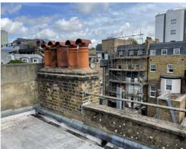
[Fig. 11] Traditional elements: Parapets, flashing, chimneys and brickwork
