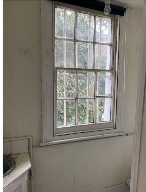
Figure 16: Original window to rear bathroom.
