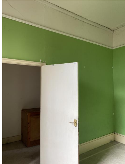
Figure 13: Modern partition and door between rear room and hallway.
