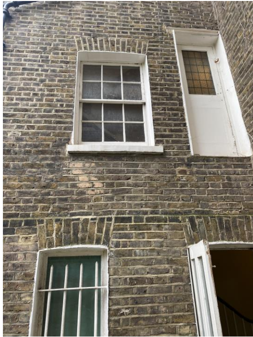
Figure 18: Historic ground floor door adjacent to original window opening.
