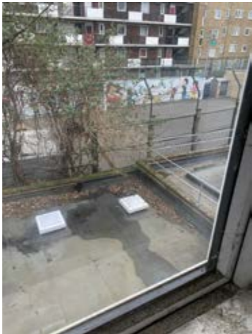
Rear view towards neighbour No.73
