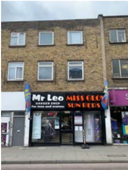
View of the front elevation
