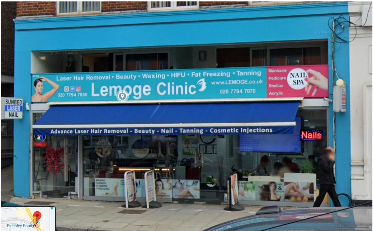
Figure 2: Streetview image showing recessed balconies above fascia sign.
