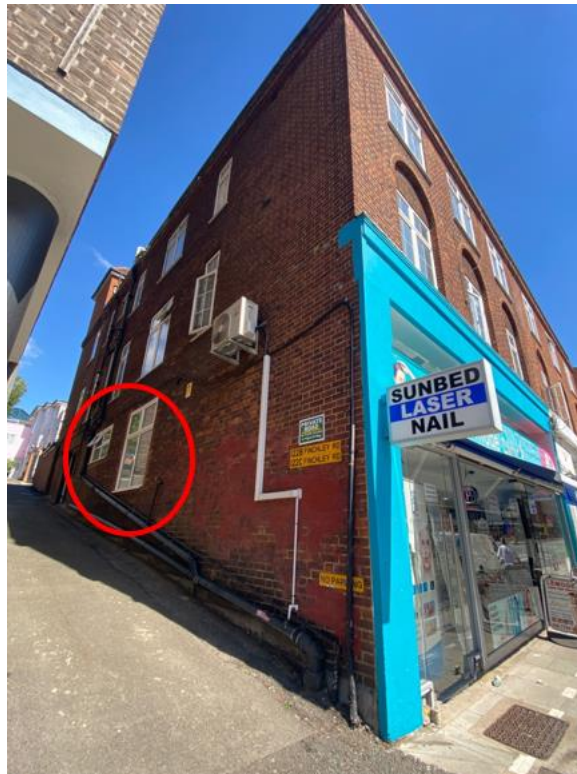
Figure 5. Site photograph showing the windows to Flat 1 on the flank elevation.
