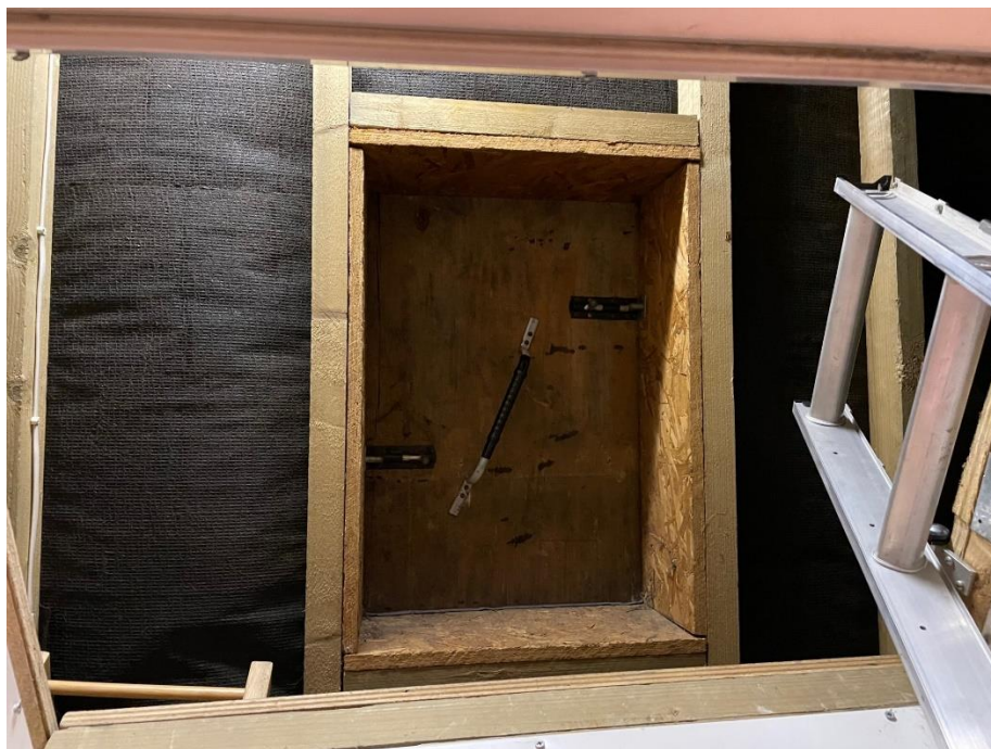
3. View of the roof access hatch taken through the loft hatch.
