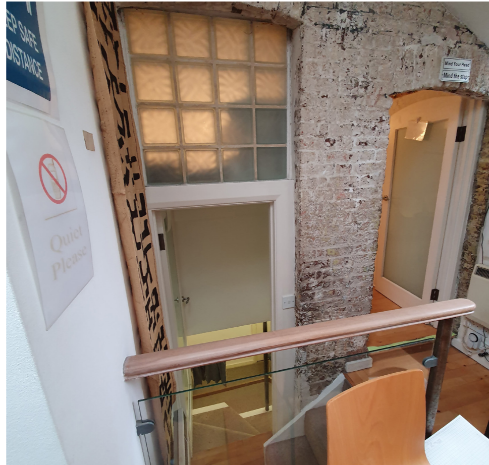
Existing opening which takes staircase down to the basement level
