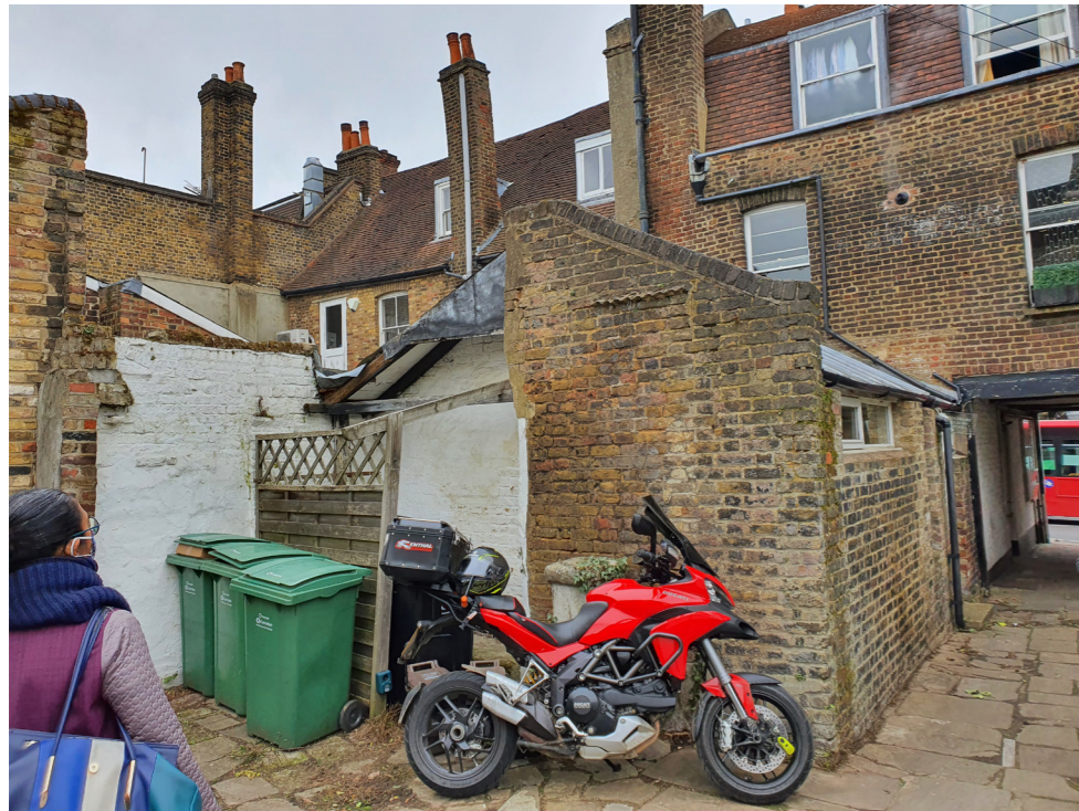
Rear single storey annexe to original building
