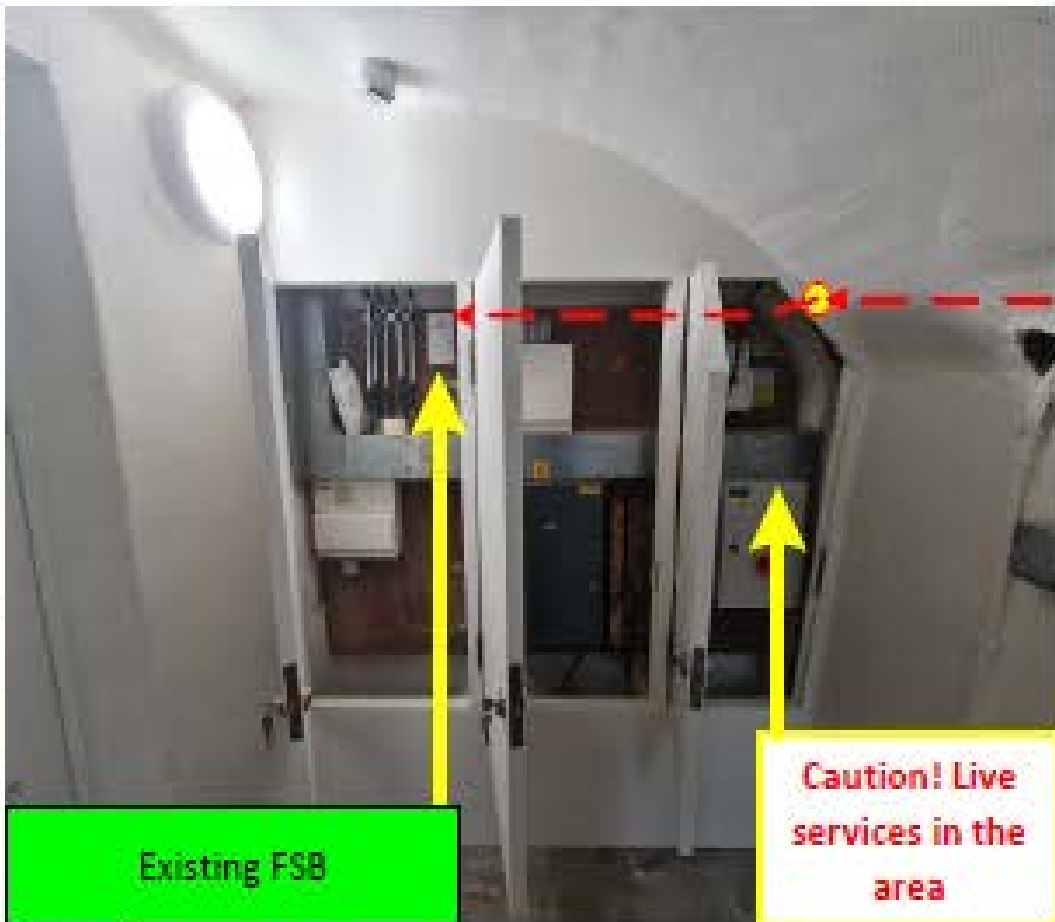
12 Multicore cable route, to existing FSB
