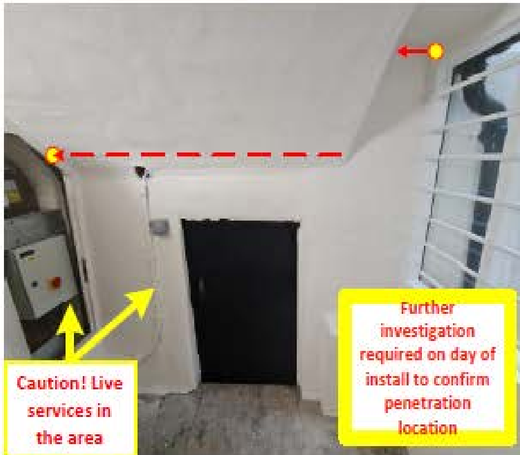
11 Multicore cable route, to existing FSB
