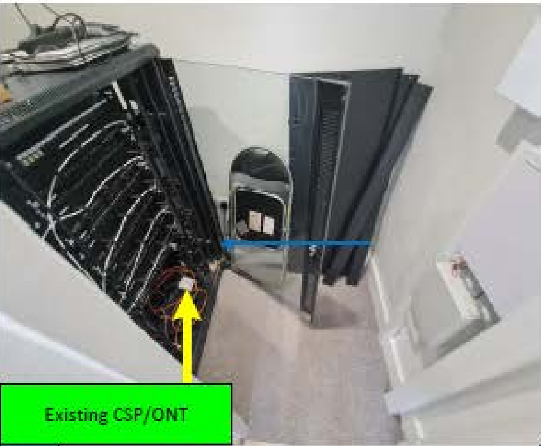
19 2f cable route, to existing CSP
