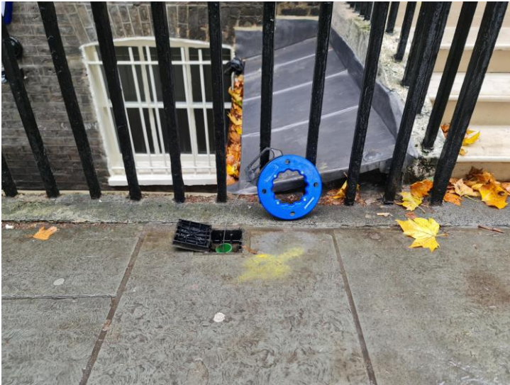
5 Picture to show toby Rodded with 5m fish tape
