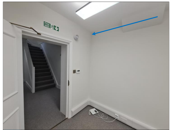
16 2f cable route, to existing CSP
