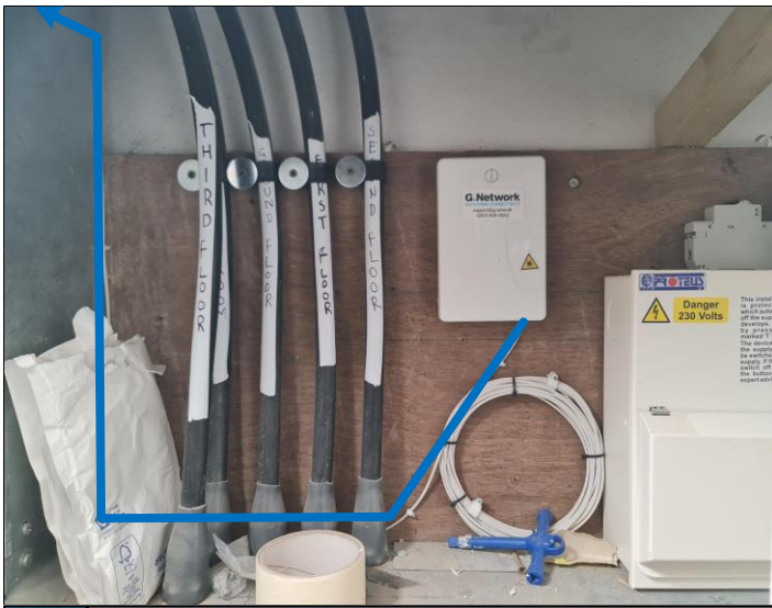
14 2f cable route, from existing FSB
