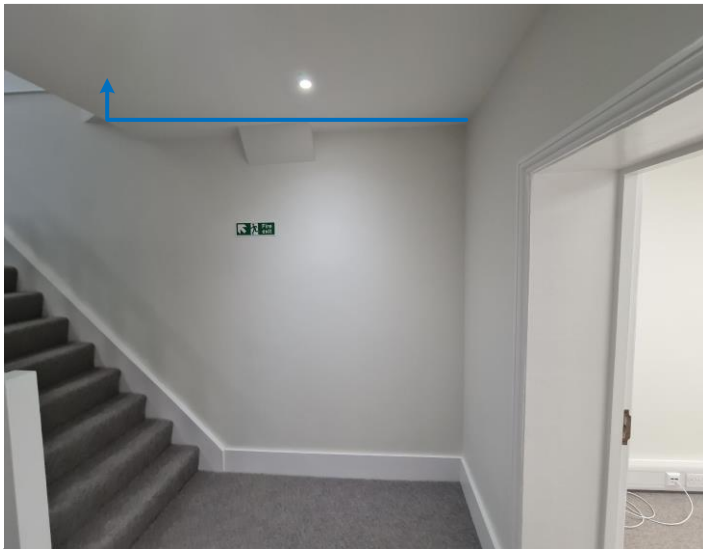
17 2f cable route, to existing CSP
