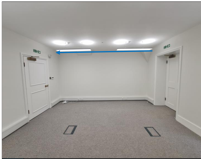
15 2f cable route, to existing CSP
