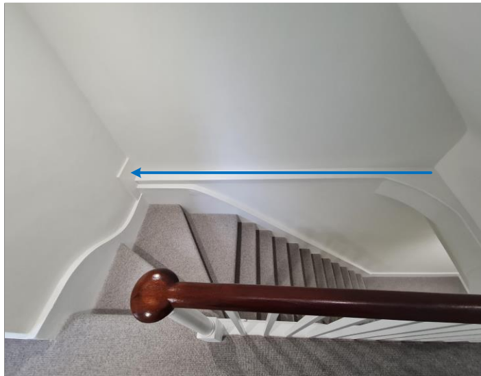
18 2f cable route, to existing CSP
