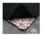
This solution is multipurpose and ideally suited to the current application. Traditional impervious barriers divert rather stop roots and may block moisture movement. Also, roots getting under such barriers can grow back to the surface. Therefore, the use of this permeable barrier stops roots either by engaging and constricting them or by chemically inhibiting them.
