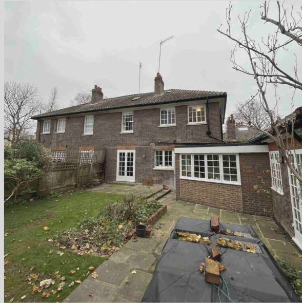
Rear Elevation Facing West
