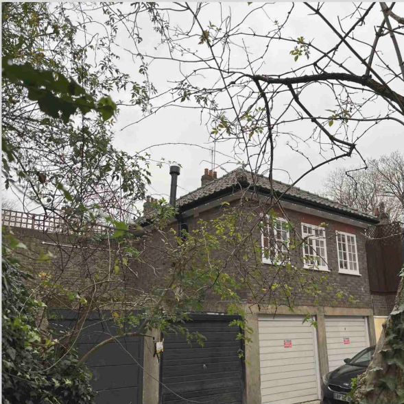
Rear/Side Elevation From Mews Facing Northwest
