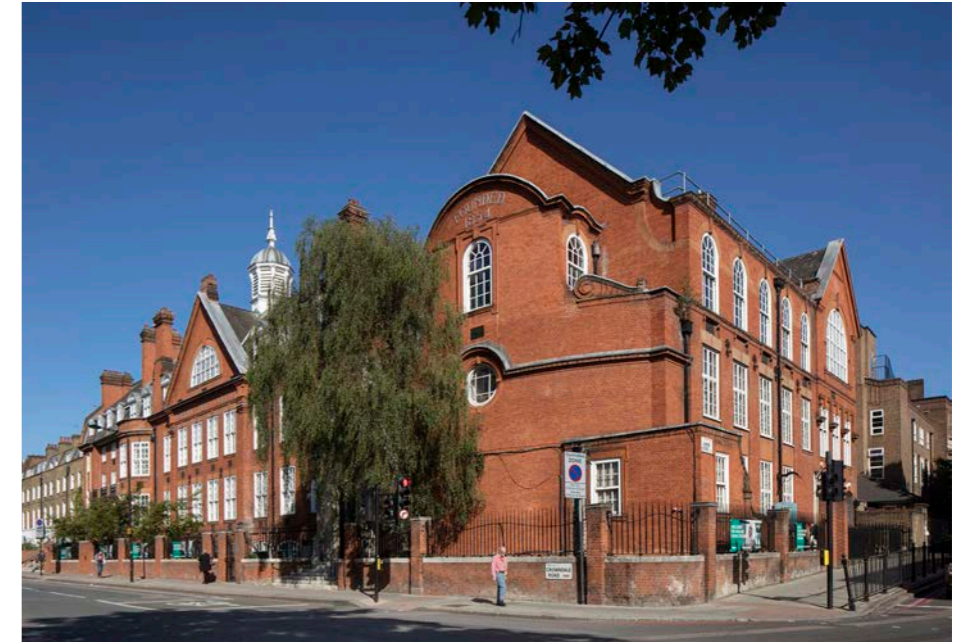
East wing of WM College, following works in 2019. The library is located in the top floor of the building
