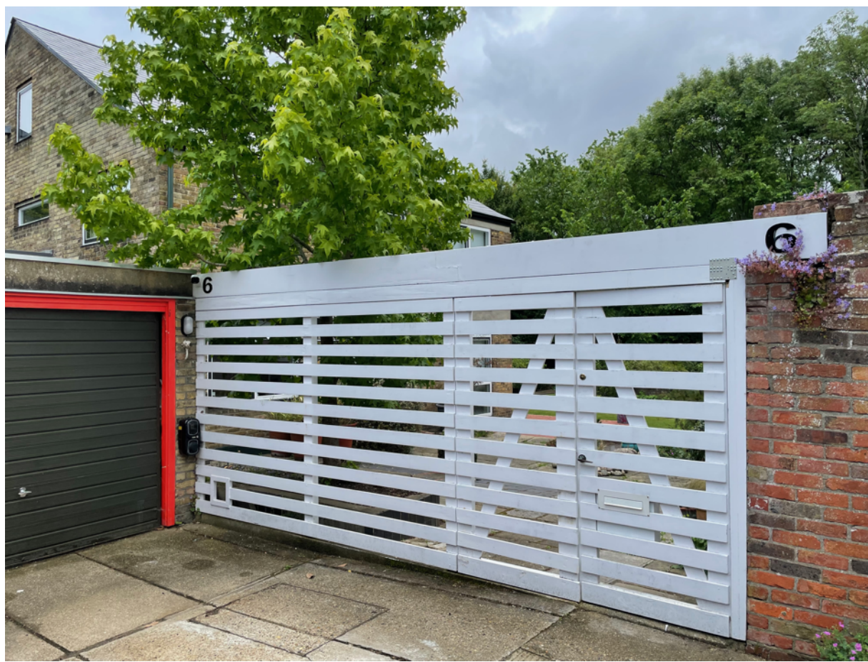
PHOTO 1: EXISTING TIMBER GATE NOT TO SCALE
