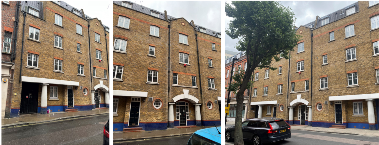
Photo 1 (above): Front elevation of Ruspini House
