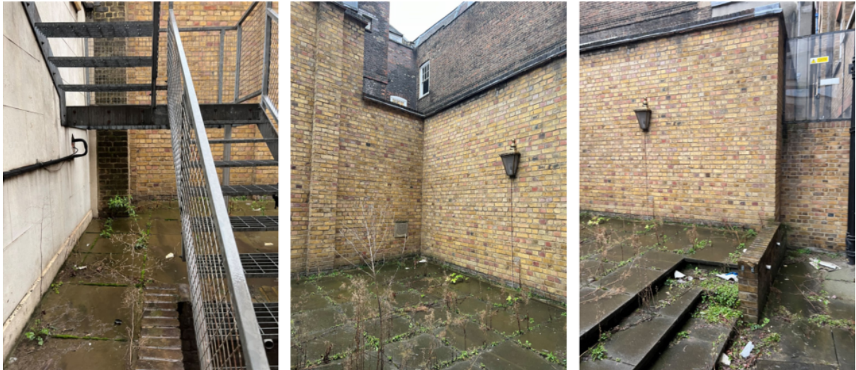
Photo 7 (above): View of area of rear courtyard where plant enclosure is proposed to be located
