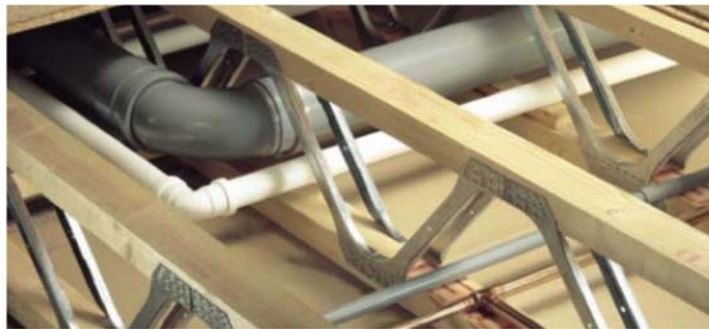
Easy joist floor construction
