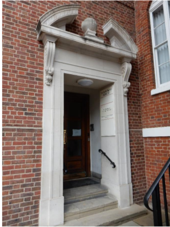
5. Existing front doorway to 10A South Square
