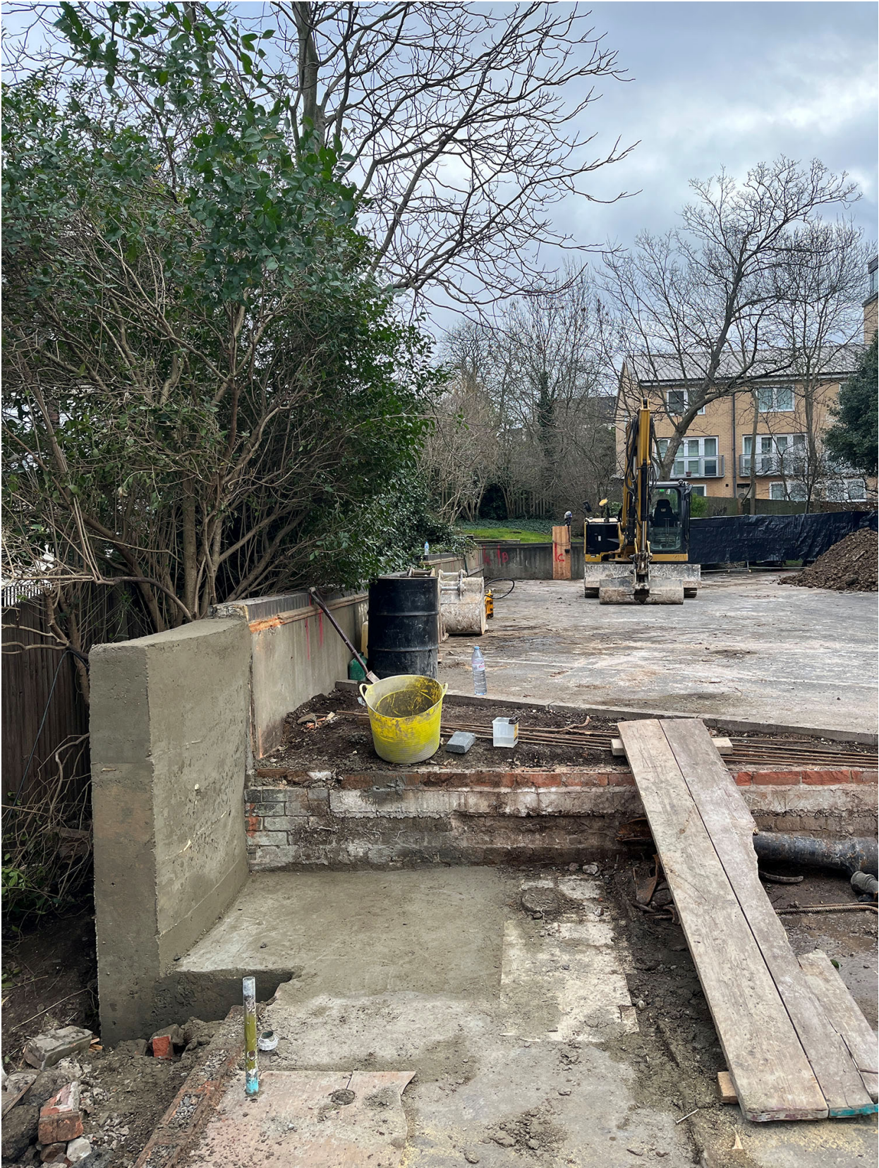
Image 4 _ 24.02.2023 _ Reinforced concrete retaining wall completed
