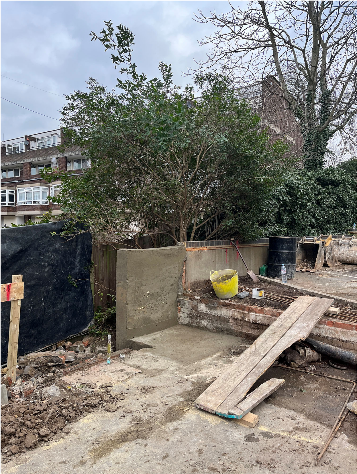
Image 5 _ 24.02.2023 _ Reinforced concrete retaining wall completed
