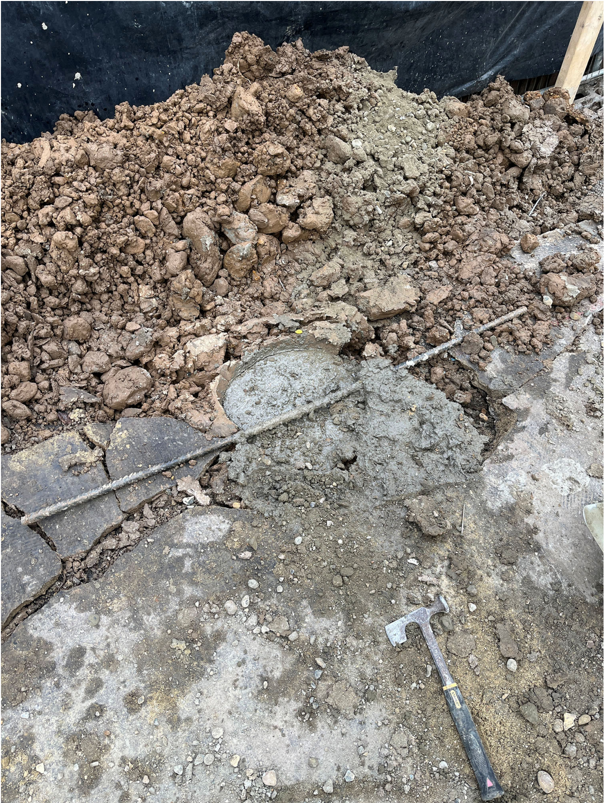
Image 7 _ 24.02.2023 _ Concrete pile completed
