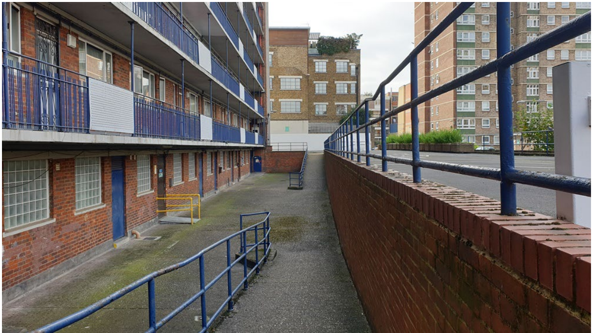
Blemundsbury northside - undercroft area
