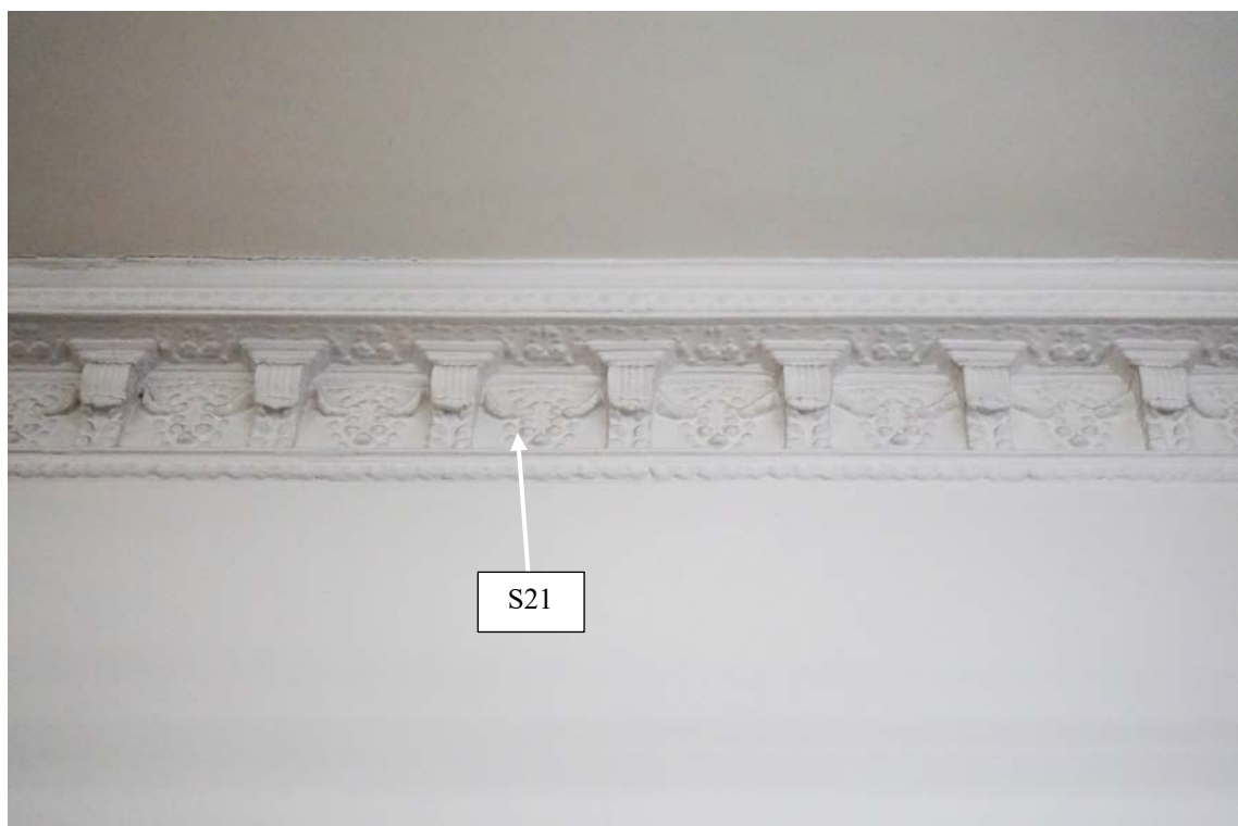
Fig. 20 Entablature on north elevation S21: berry & ground
