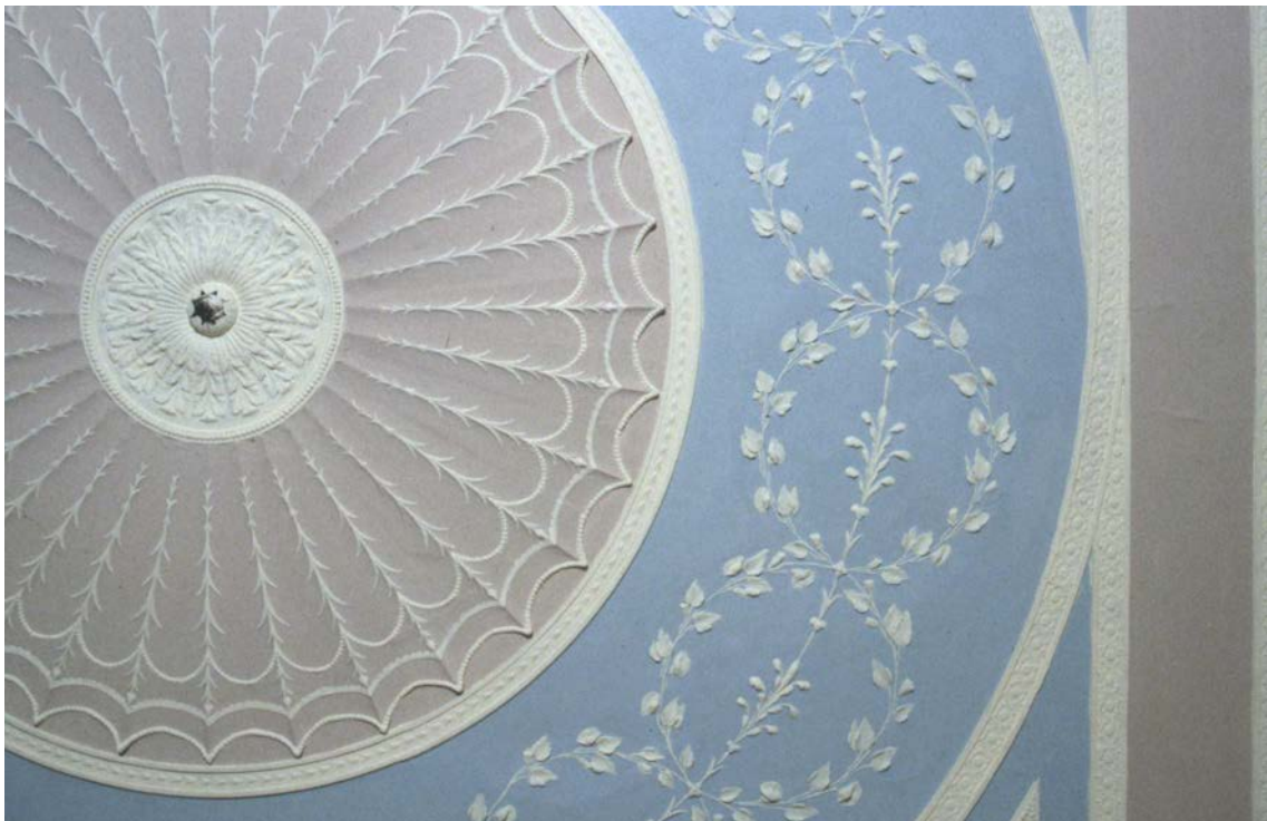
Plate 4 Emulation of lead white relief with Prussian blue and vermillion tinted flatwork
