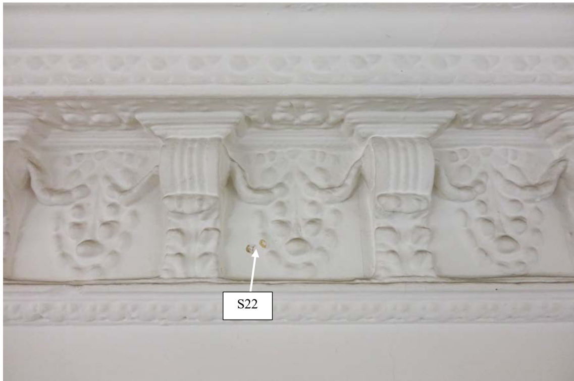
Fig. 21 Entablature on west elevation S22: berry/ground
