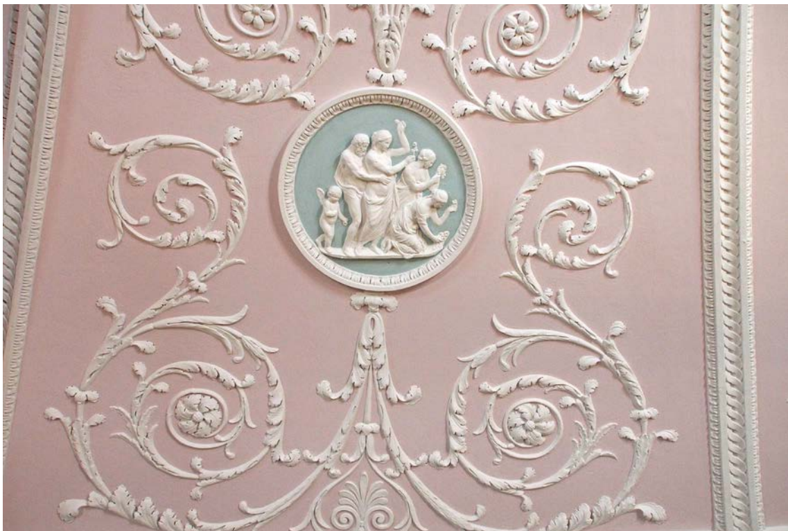
Plate 2 Emulation of Lead white relief and vermillion and red lake tinted flatwork
