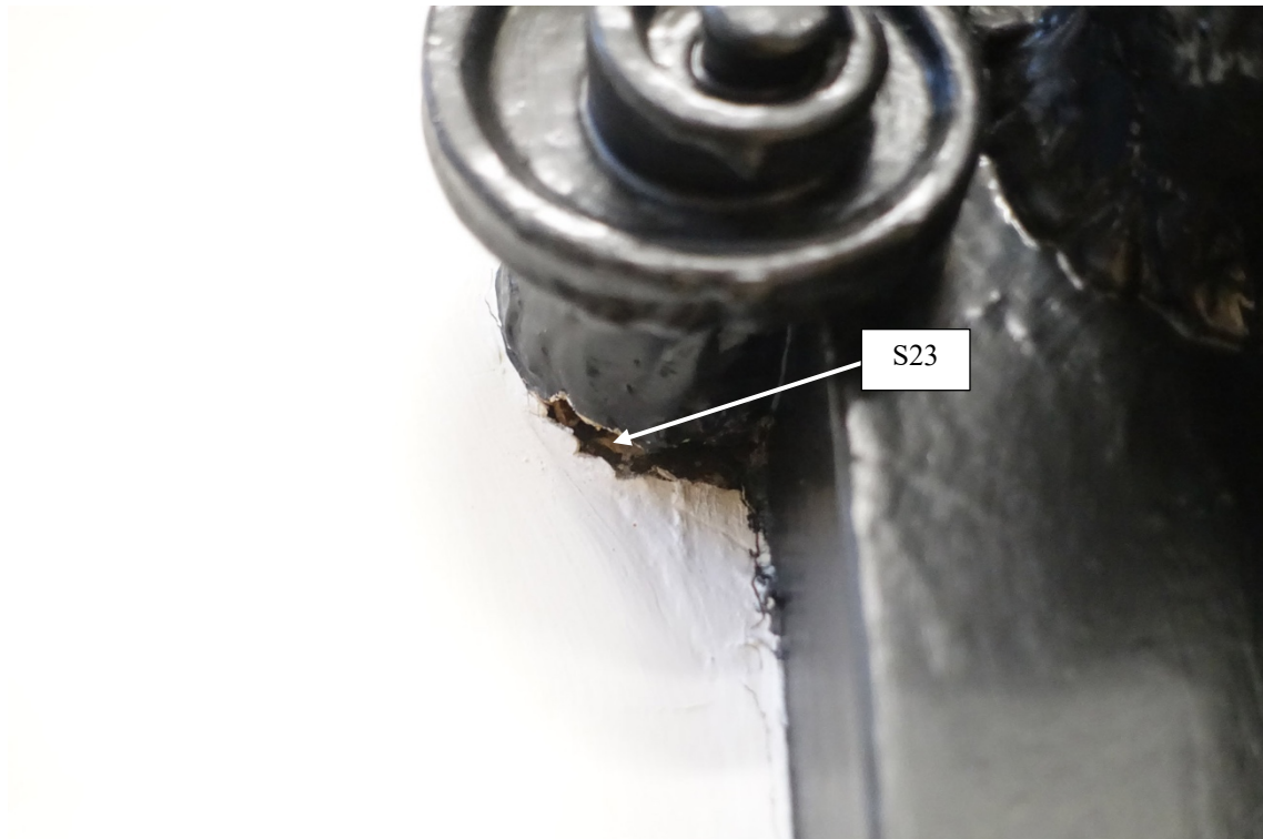
Fig. 23 Sample from beneath volute of dexter side hard against wall
