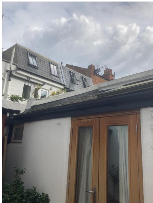
4. Existing pitched roof with flat apex on existing rear extension
