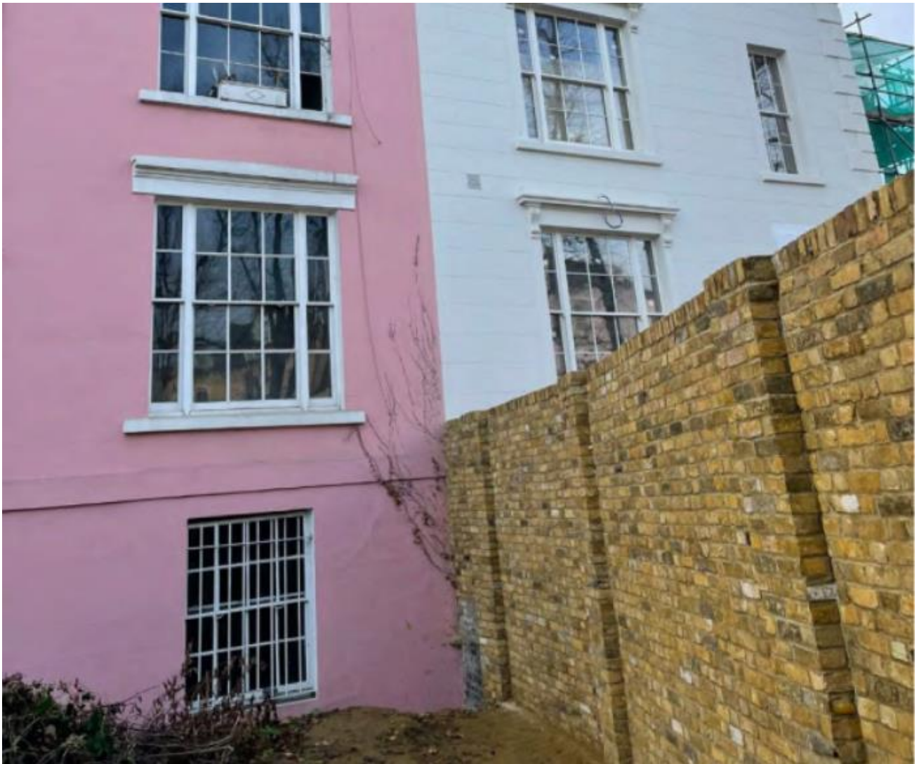
5. Existing garden boundary wall to the rear between No 5 and No 6 Albert Terrace
