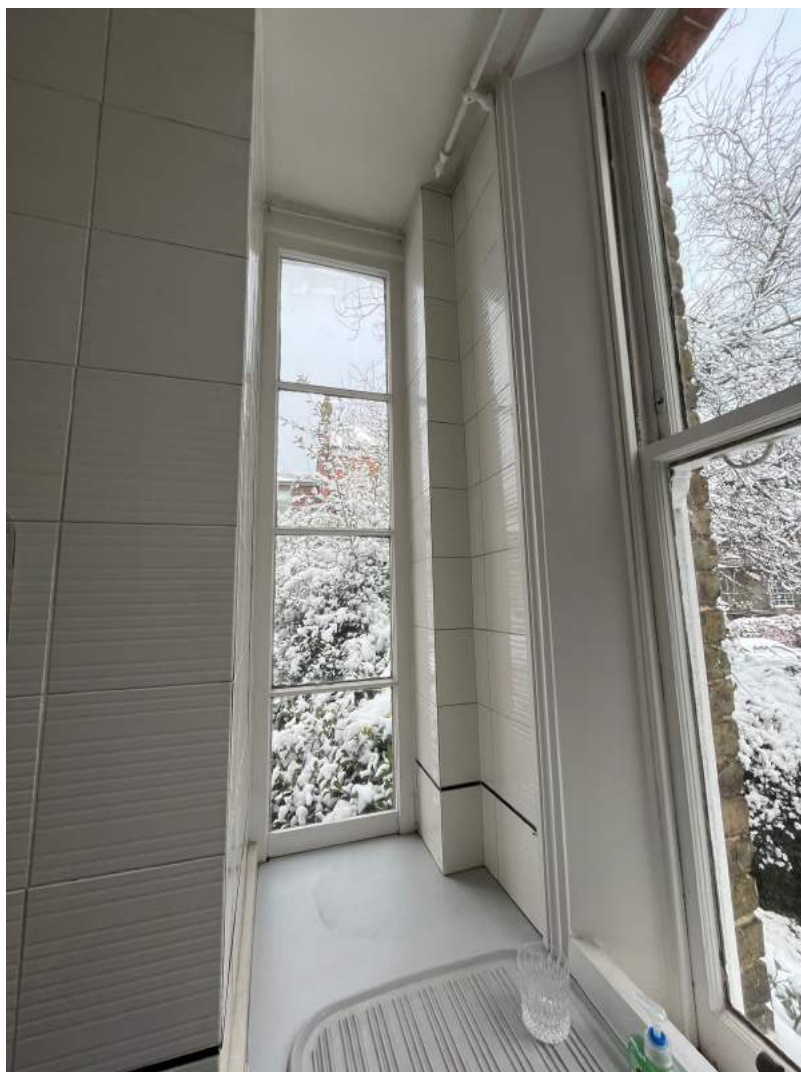
Existing fixed single glaze window in kitchen
