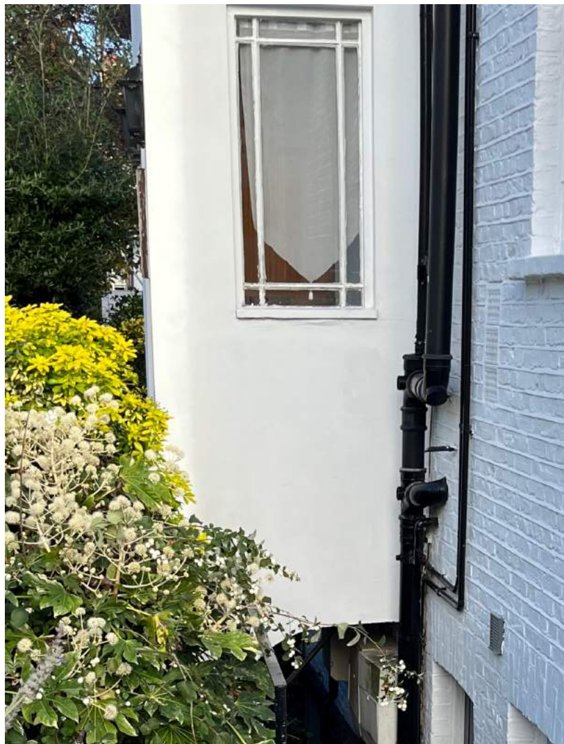
Existing fixed single glazed windows by main entrance (external)
