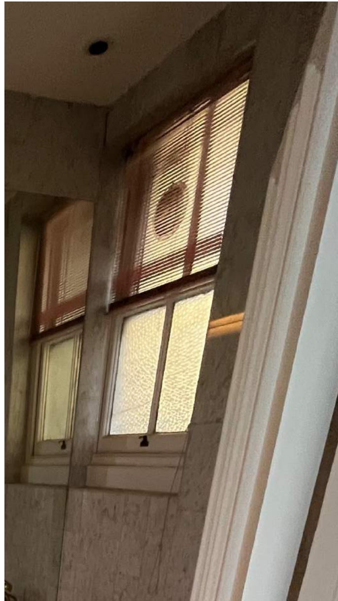
Existing sash single glaze window in bathroom
