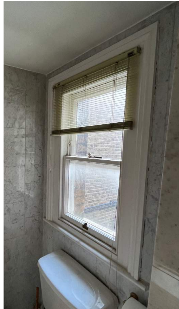
Existing sash single glaze window in ensuite
