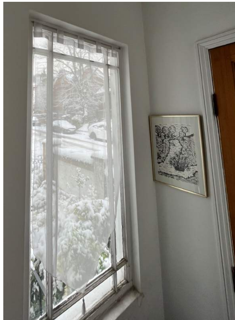
Existing fixed single glazed windows by main entrance (internal)
