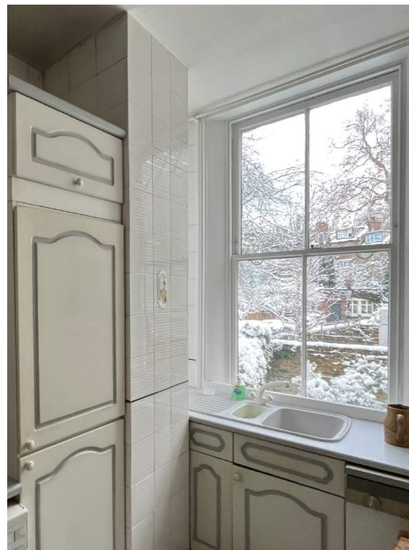
Existing sash single glaze window in kitchen
