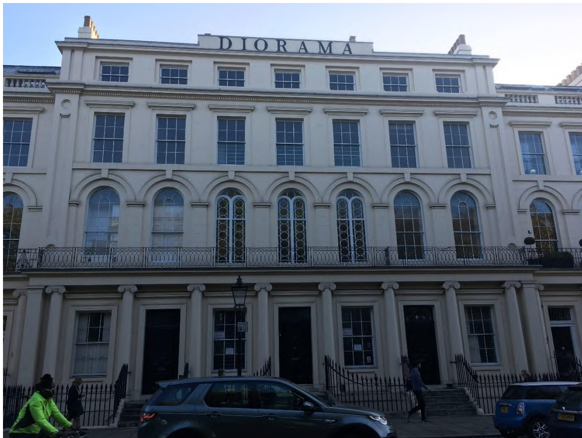
Figure 39 The Park Square East elevation of nos. 17-19, which projects forward of the rest of the terrace. No. 18 occupies the central three bays. The windows at first floor were inserted in the 1850s. The original arrangement of entrance door and flanking windows was reinstated in the 1990s.
