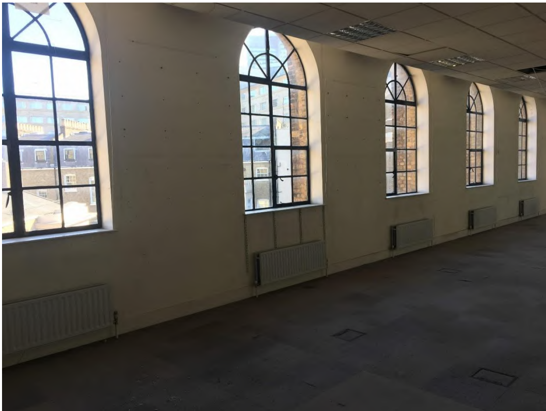
Figure 43 The suspended ceiling in 1990s open plan office cuts across the tops of the 1929/30 windows in 1850s arched openings at second floor.
