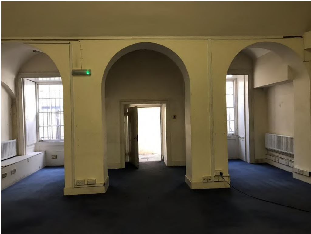
Figure 54 Looking towards the front area of no. 18. The thick front wall with deep door and window reveals is visible. The arches in front are beneath steps in no. 18's entrance which were originally constructed in the 1850s.
