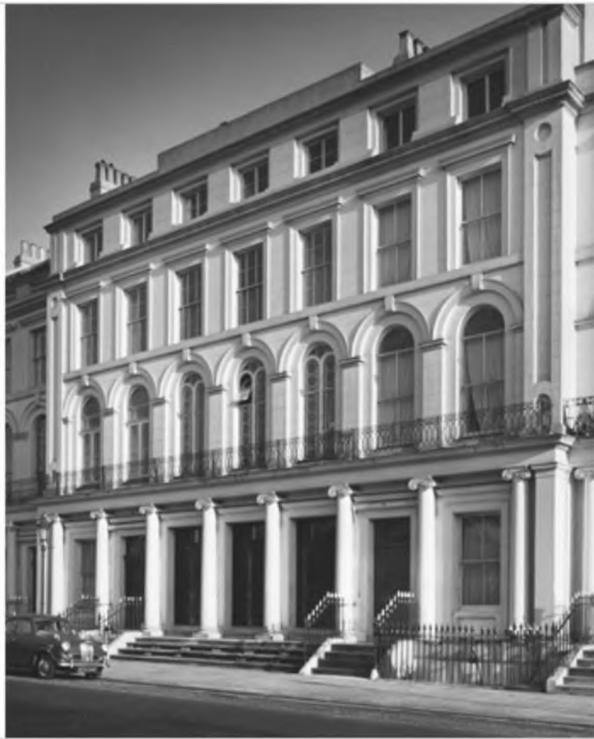
Figure 21 1962 photograph of the front elevation of 17-19 Park Square East. The 1850s alteration to the entrance of no. 18 (creating three doorways instead of one) is still in place, although the central and left hand door were redundant by this point as the Institute had inserted an additional floor inside. RIBA Pix ref no.: RIBA5342.
