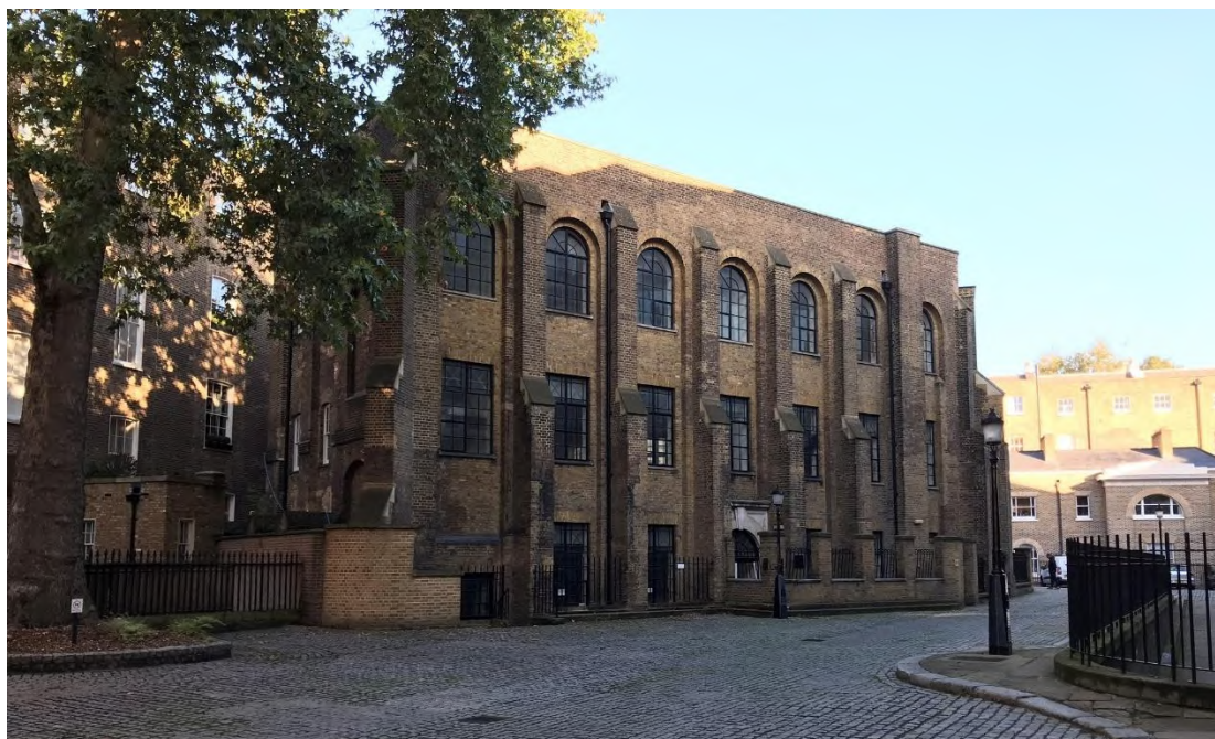
Figure 40 South-east elevation of the Diorama building in Peto Place. The form of the building dates from the 1820s, the arched openings and buttresses were part of the 1850s chapel conversion, the metal-framed windows and stone door surround were inserted in 1929/30.
