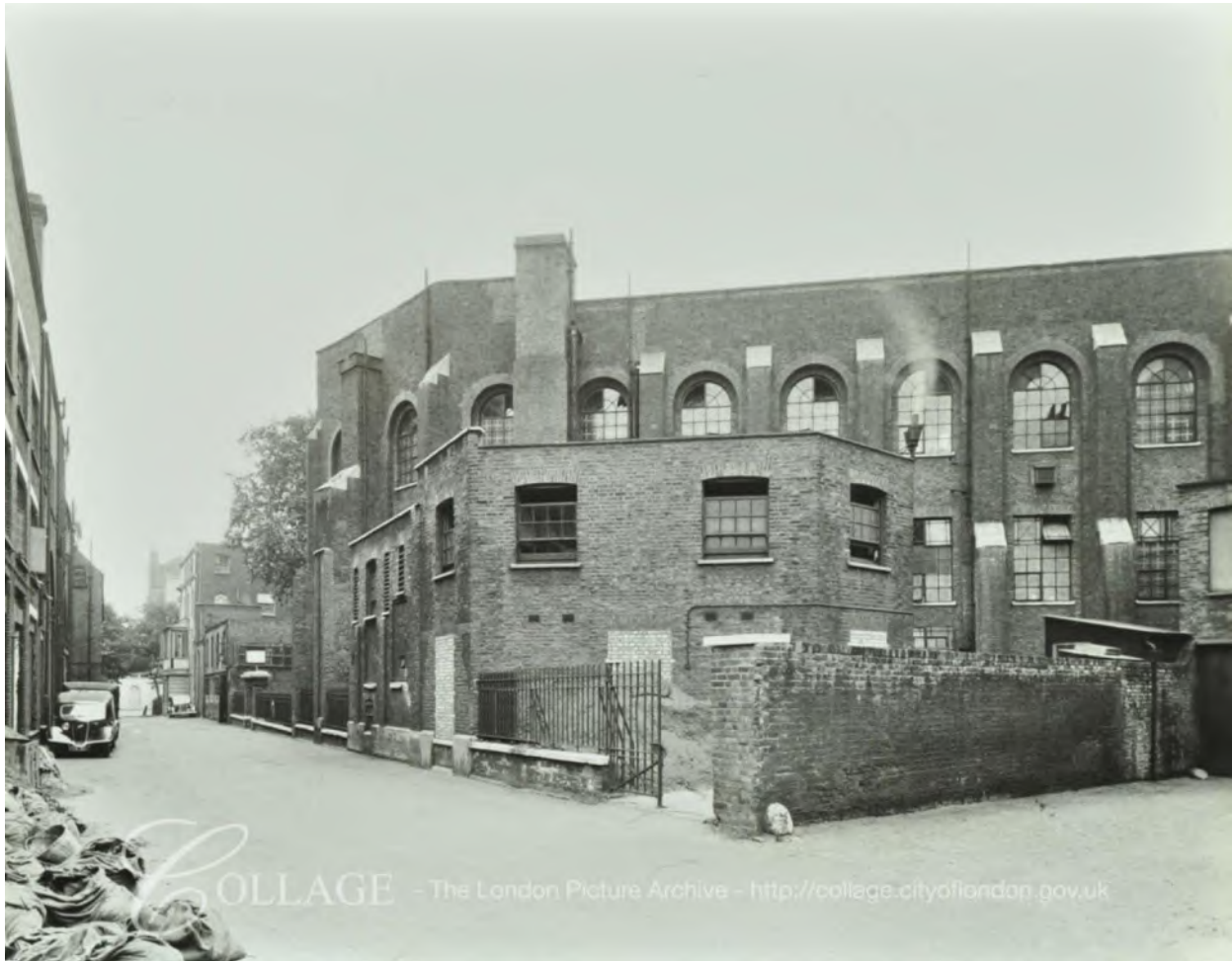
Figure 18 Photo of the rear of the Diorama building, Peto Place, 1941. The rear wall has a raised parapet. LMA Collage Record No. 113747.
