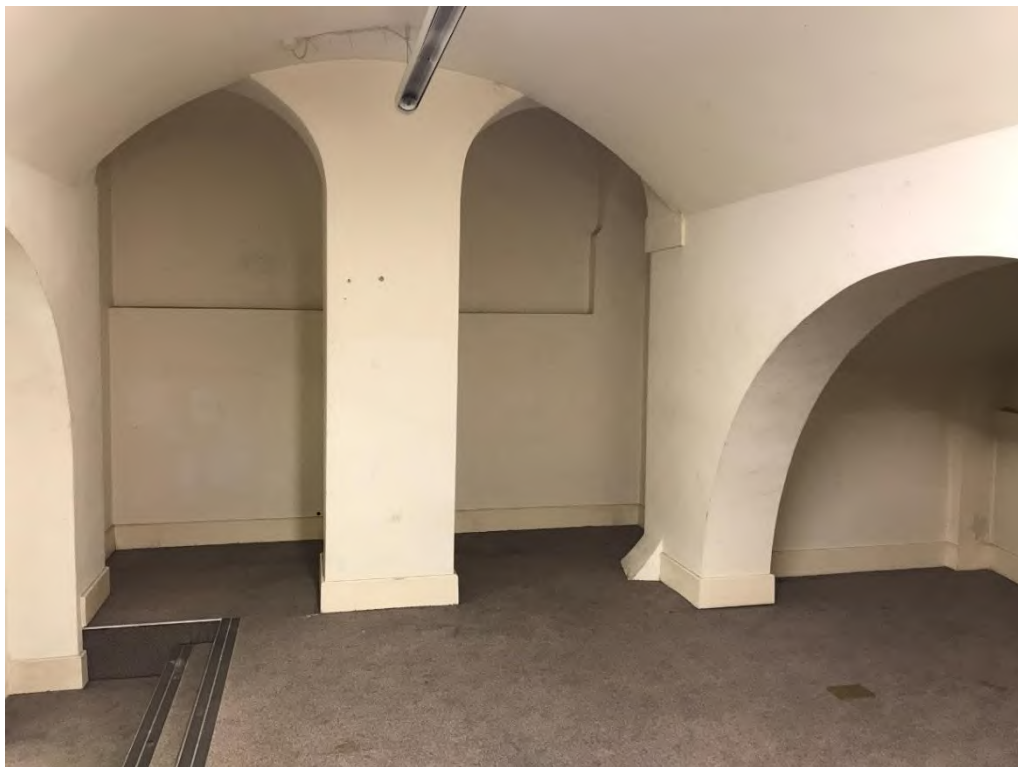
Figure 53 Basement of the front part of no. 18. The arches were constructed to support the 1850s chapel steps, screen and staircases.
