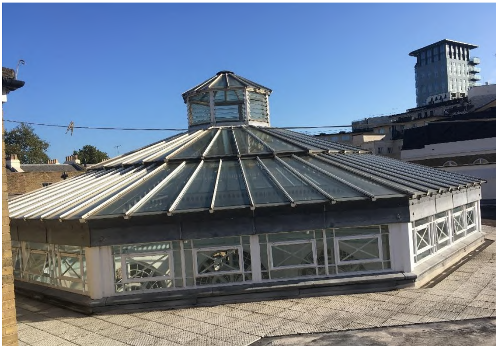
Figure 49 Octagonal lantern over the lightwell through the Diorama building. 1990s replacement of 1929/30 structure.
