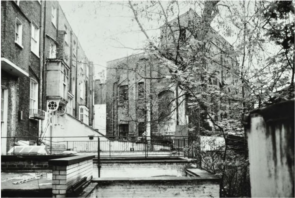
Figure 25 '20-24 Park Square East: rear elevations', 1985. The south elevations of the Diorama building are partially visible in this photo, showing that windows had been inserted in the originally blank arches of the flank wall. The plant and tank rooms are also prominent features on the roof. LMA Collage Record No.: 106298.
