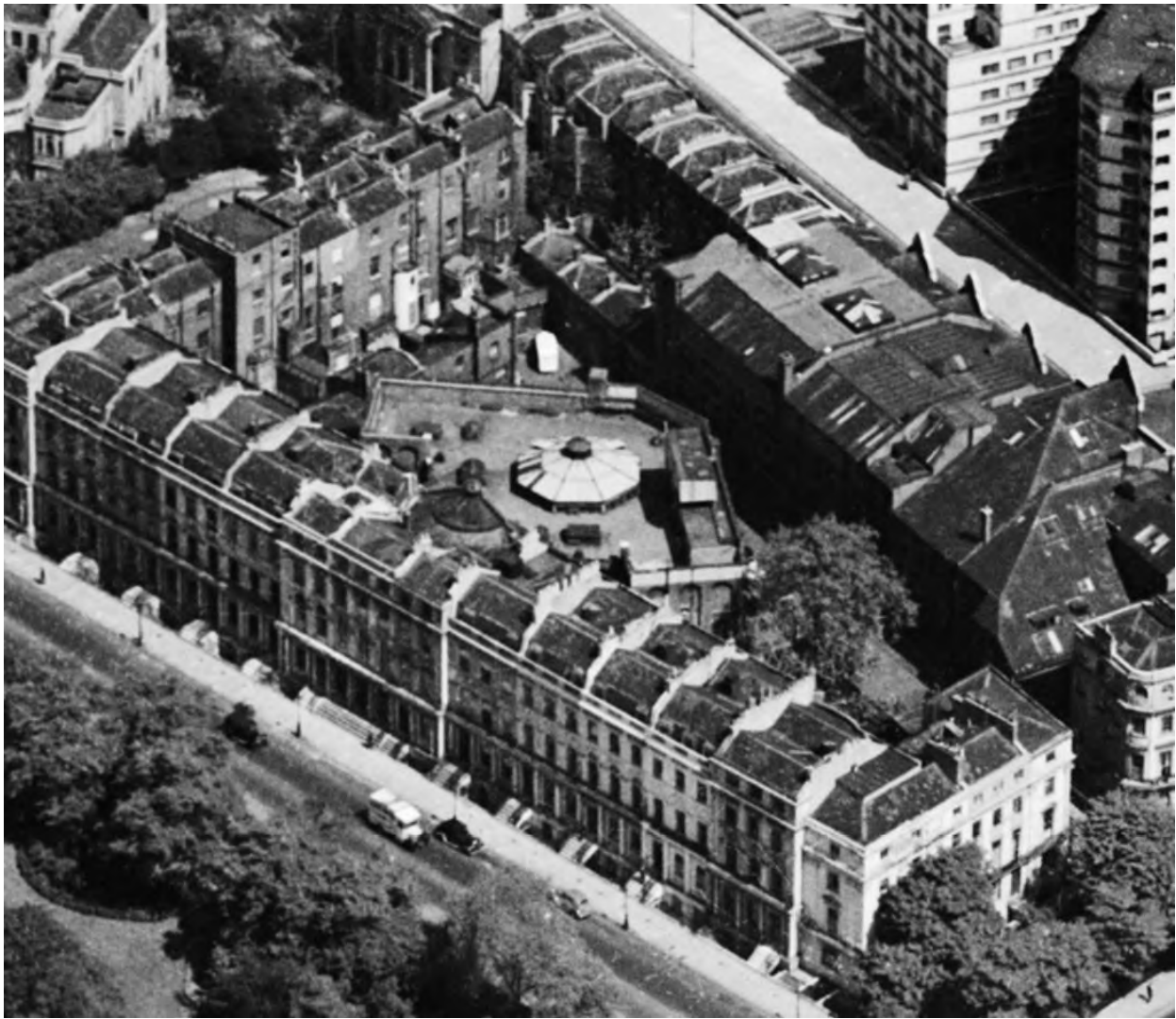
Figure 19 Aerial photograph from the south-west, 1946. The changes to the roof undertaken as part of the Diorama building's conversion to rheumatism clinic are visible and include the bisection of the Diorama's conical rooflight, construction of flat roof in place of the chapel's hipped roof, construction of a larger octagonal rooflight, construction of plant and tank rooms on the roof. Britain From Above, ref: EAW000542.
