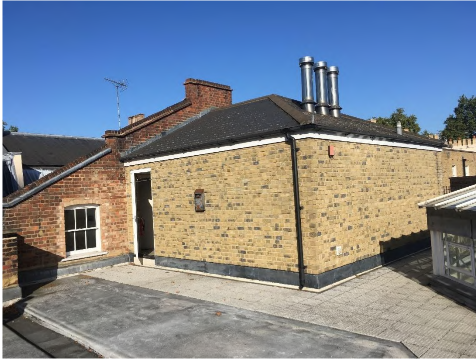
Figure 50 1929/30 gable (in red brick) terminating the conical rooflight over the Diorama's saloon. The yellow brick structure dates from the 1990s conversion or later.
