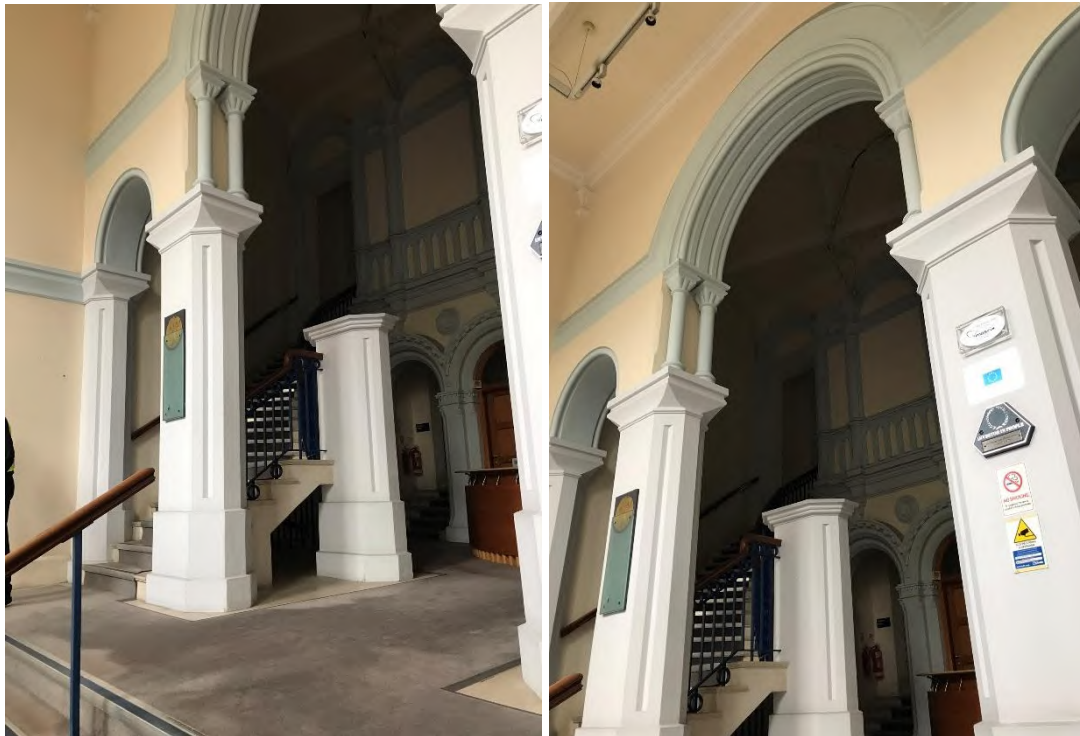
Figure 51 Screen at the front of the chapel vestibule. The structure of the screen dates from the 1850s conversion, the fibrous plaster enrichment dates from the 1990s refurbishment. The staircase and standalone column also date from the 1990s.
