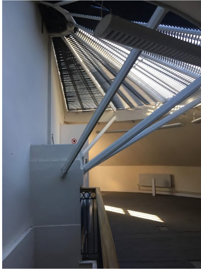
Figure 47 The remaining half of the conical rooflight over the Diorama's saloon. Although the fabric has been renewed and the timber supports radiate from the 1850s structure, the form of the rooflight is believed to be consistent with the Diorama's roof.
