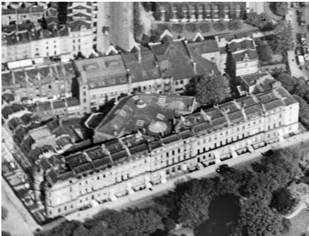
Figure 8 Detail of aerial photograph from the north-west, 1926. The roof form of the 1850s chapel is evident, including hipped roof over the wings of the Diorama building, octagonal light/louvre over the chapel, and the Diorama saloon's conical rooflight. Britain From Above ref: EPW015723.
