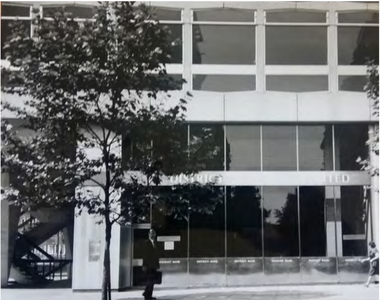
18C Kingsway block, ground floor elevation, 1969 (RIBA Photographs Collection)
