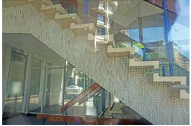
43A Southern staircase treads, Kingsway block (Insall)
