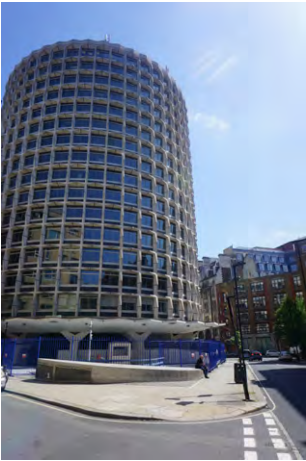
45 Tower block exterior (Insall)
