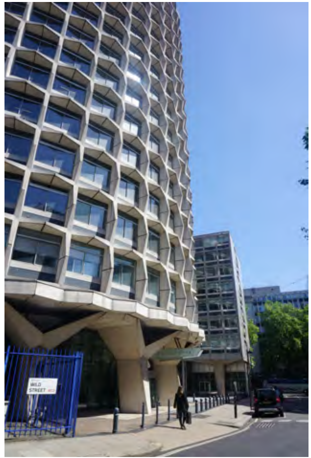
46 Ground floor pilotis, tower block (Insall)
