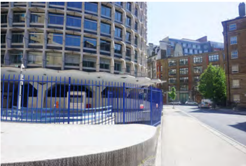
35A Modern railings to rear of site (Insall)
