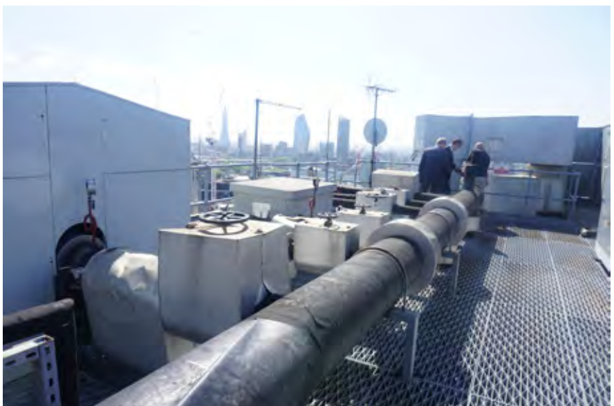
49C Tower block roof plant (Install)
