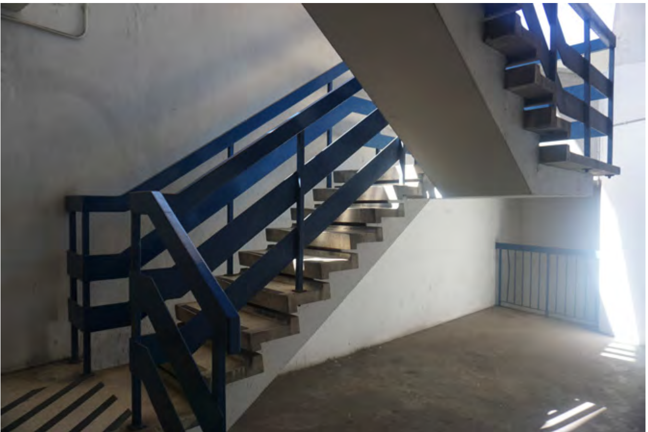
47C Original ramp access stairs (Insall)
