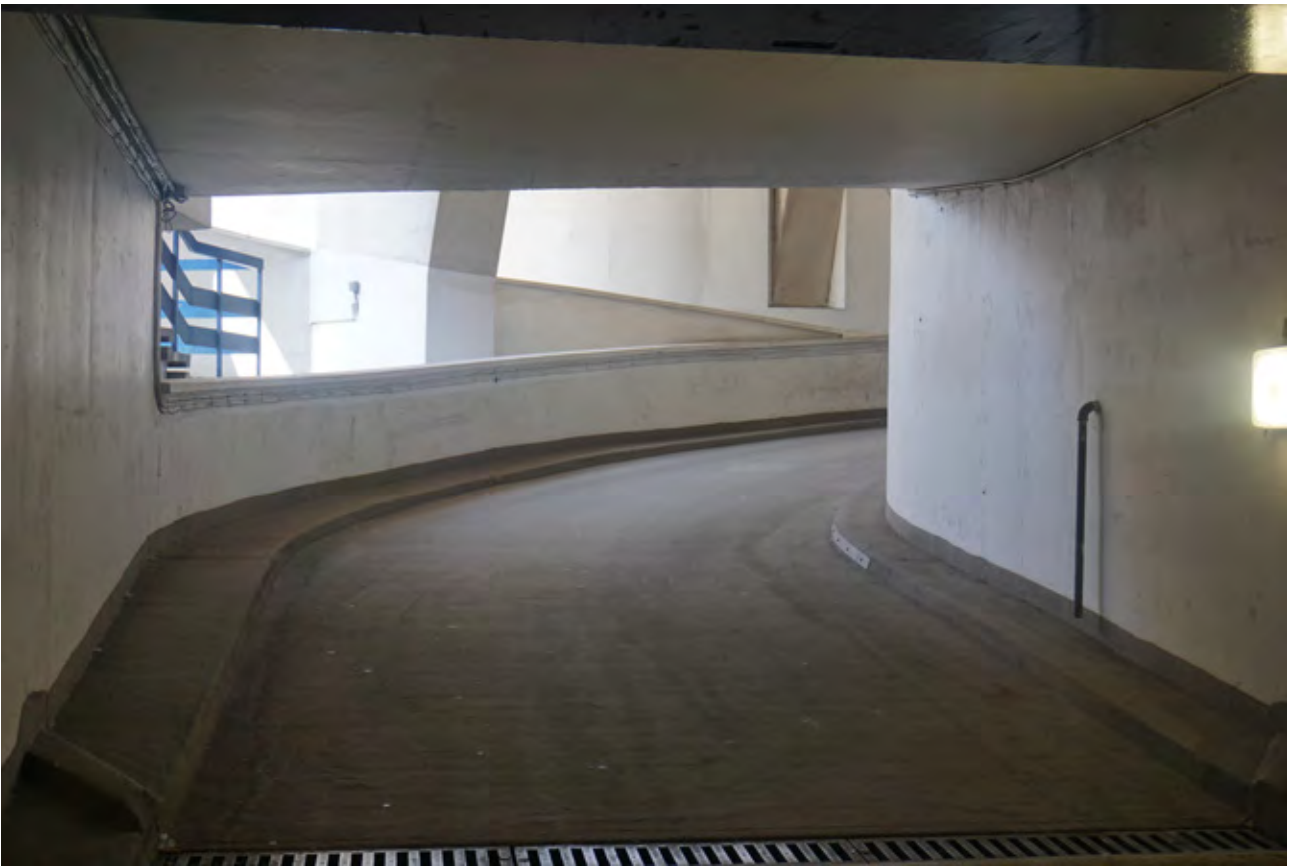
47B Original garage ramps (Insall)
