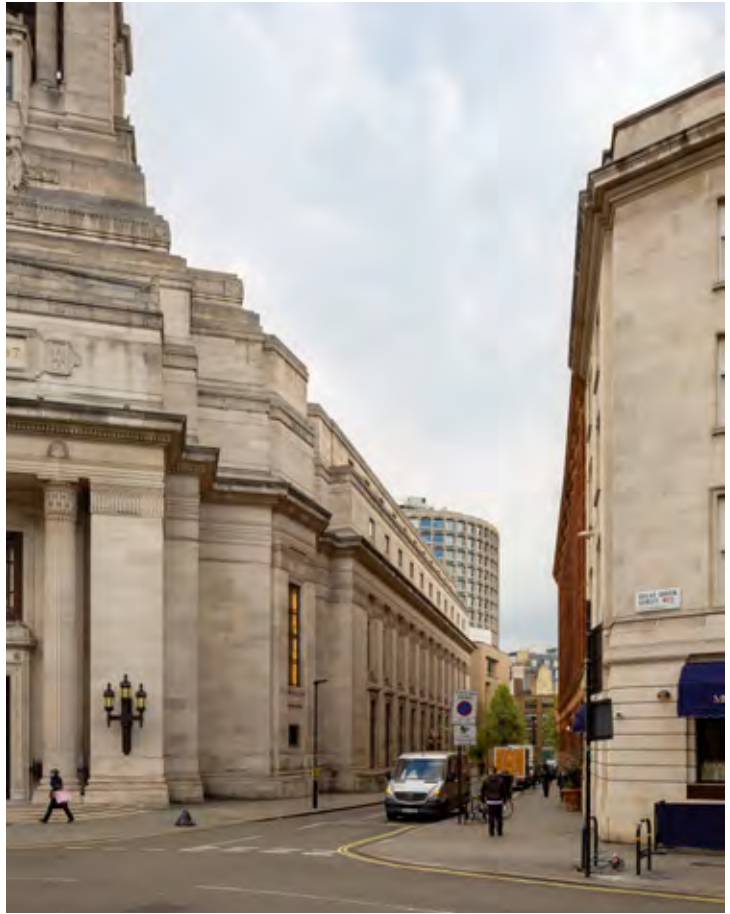
65A Existing view from corner of Great Queen Street & Wild Street (Squire & Partners)
