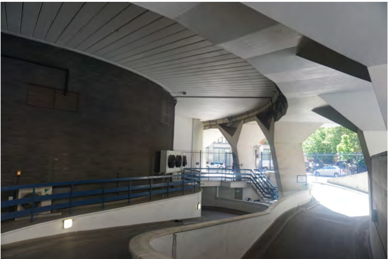
47A Original garage ramps (Insall)
