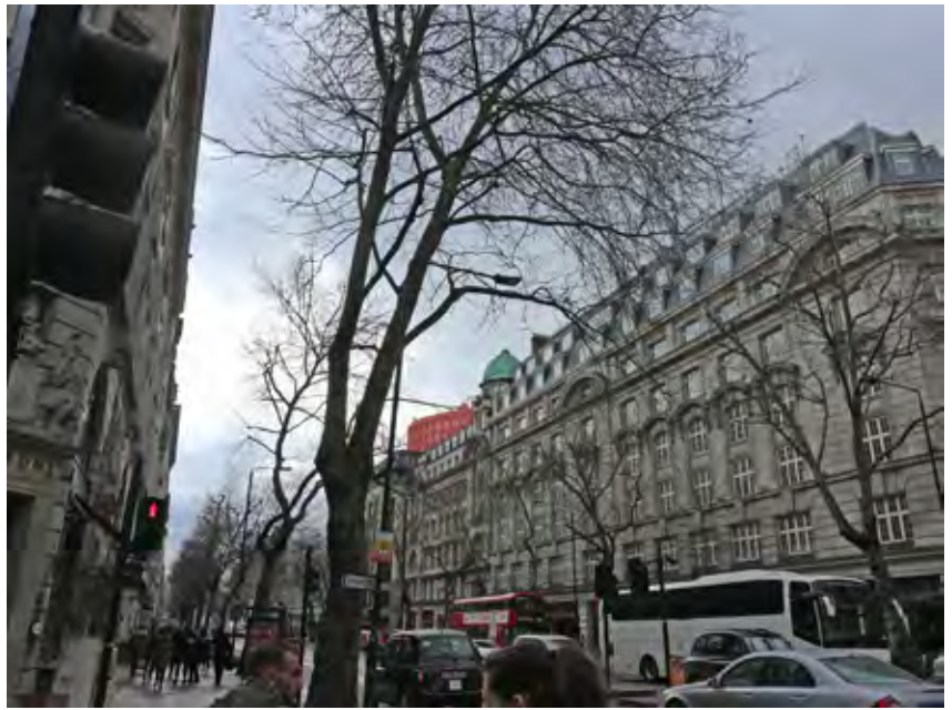
31A CAA House tower visible from Kingsway (marked in red) (Insall)
