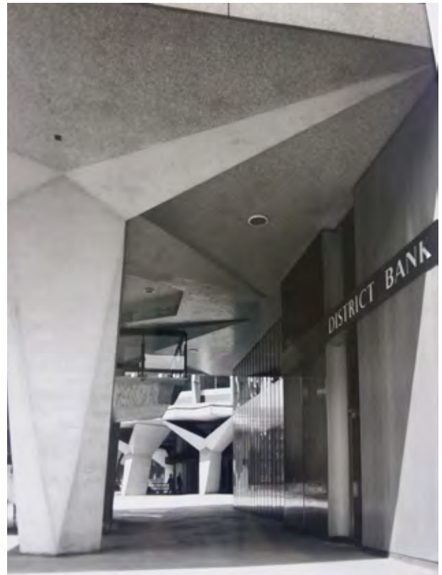
18B 1969 photograph of Kingsway block, looking west (RIBA Photographs Collection)
