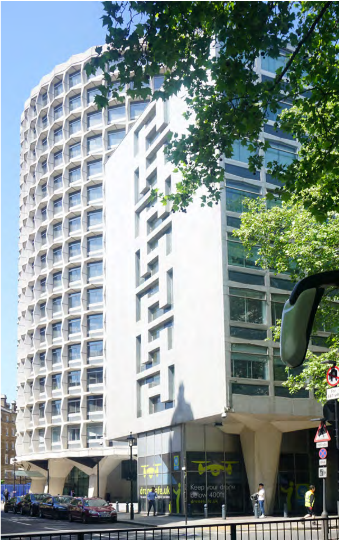
40A Kingsway block southern return elevation (Insall)
