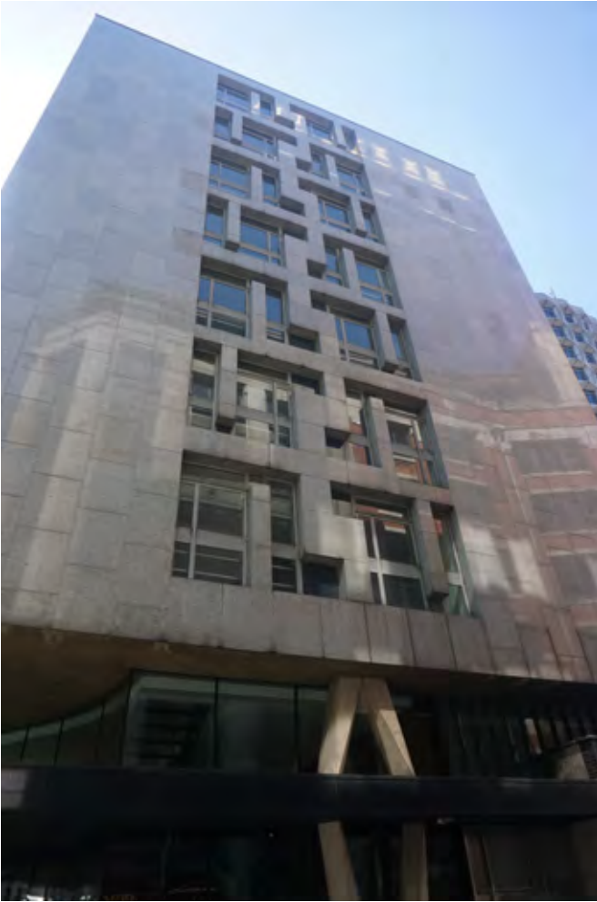
38 Kingsway block side elevation, upper floors (Insall)
