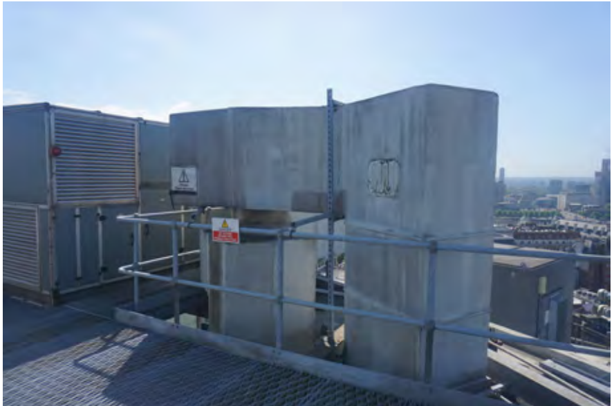
49B Tower block roof plant (Install)
