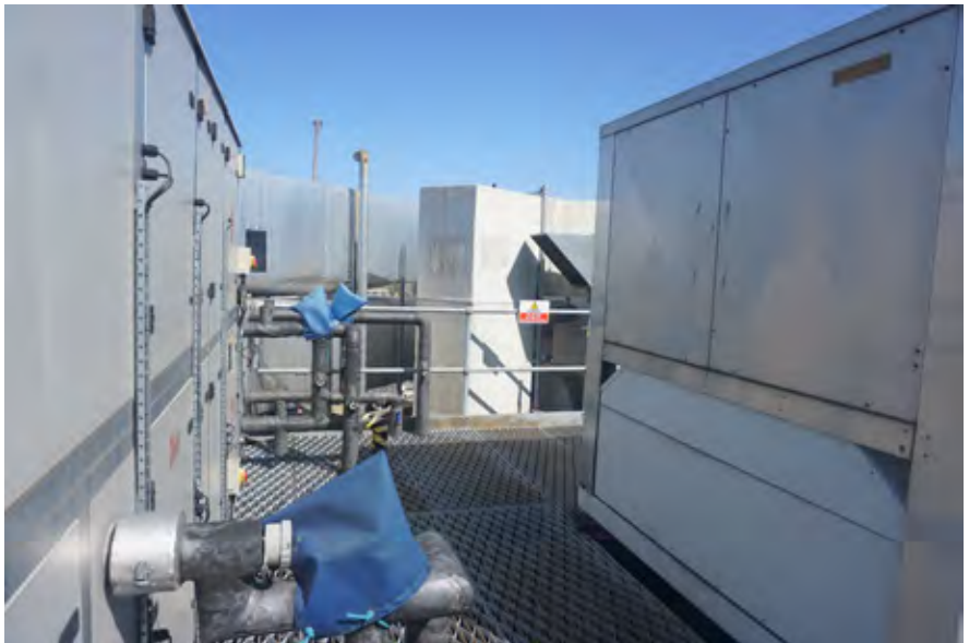
49A Tower block roof plant (Install)
