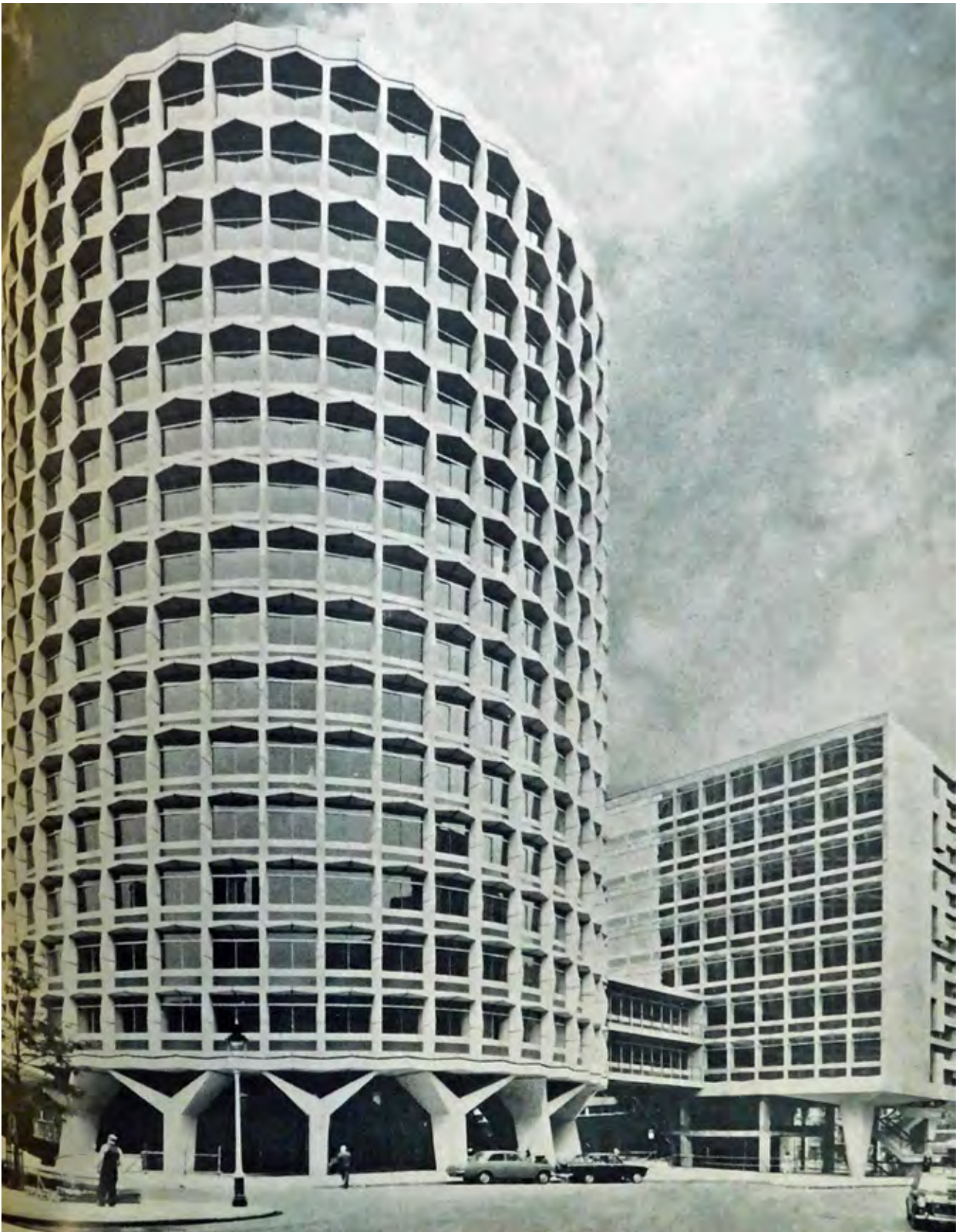
27A Space House looking east, 1968 (RIBA Library)
