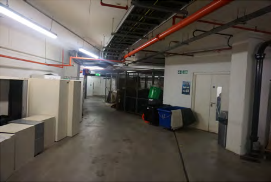
55 Tower block, underground garage area (Insall)
