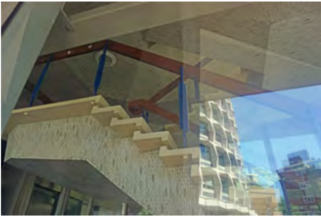
43B Southern staircase, Kingsway block (Insall)
