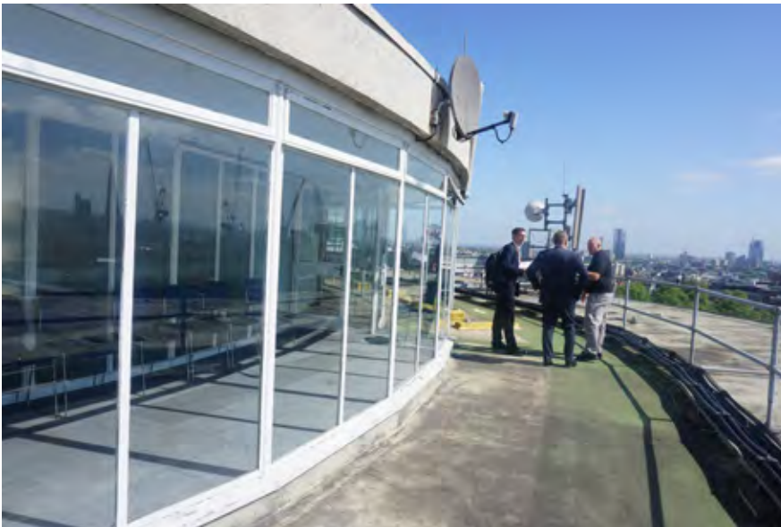
51A Tower block roof enclosure (Insall)
