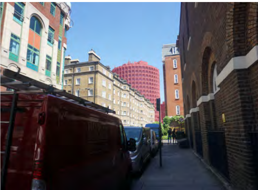
34A CAA House visible from west (marked in red) (Insall)
