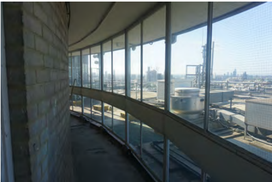
51B Tower block roof enclosure (Insall)
